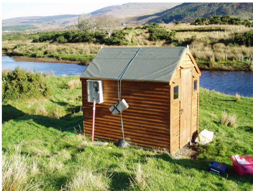
Figure 3.9 The Black River station: the timber shed housing the pump, flow cell and electronics.
