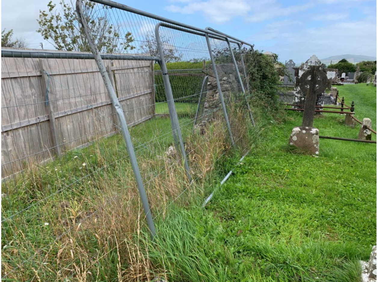
Figure 1-1: Collapsed Wall
