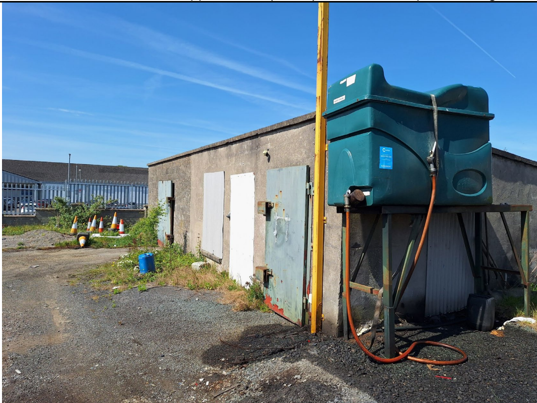
Image 14: View of 1 No. 1,200-litre approx. AST (diesel) adjacent to storage shed at western site boundary, facing west. No bunding, ground staining observed.
