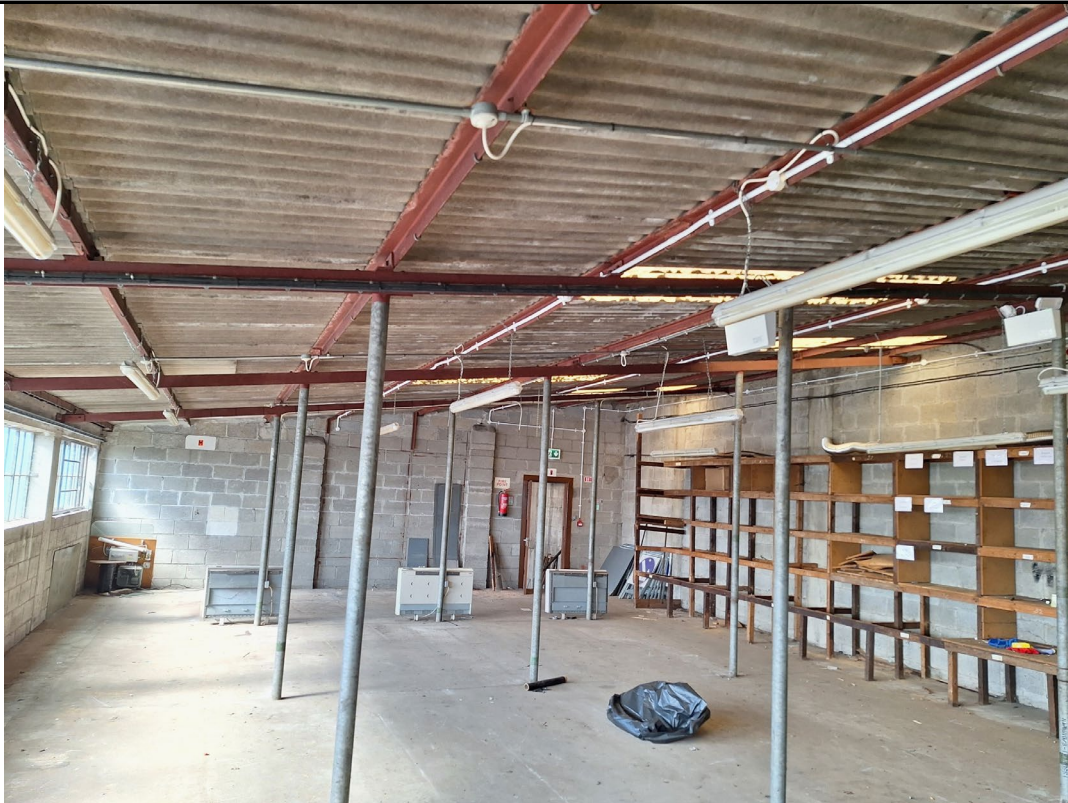
Image 27: View of small stores room located on south side of main workshop, concrete flooring, block walls, steel roof beams supported by narrow diameter circular metal
