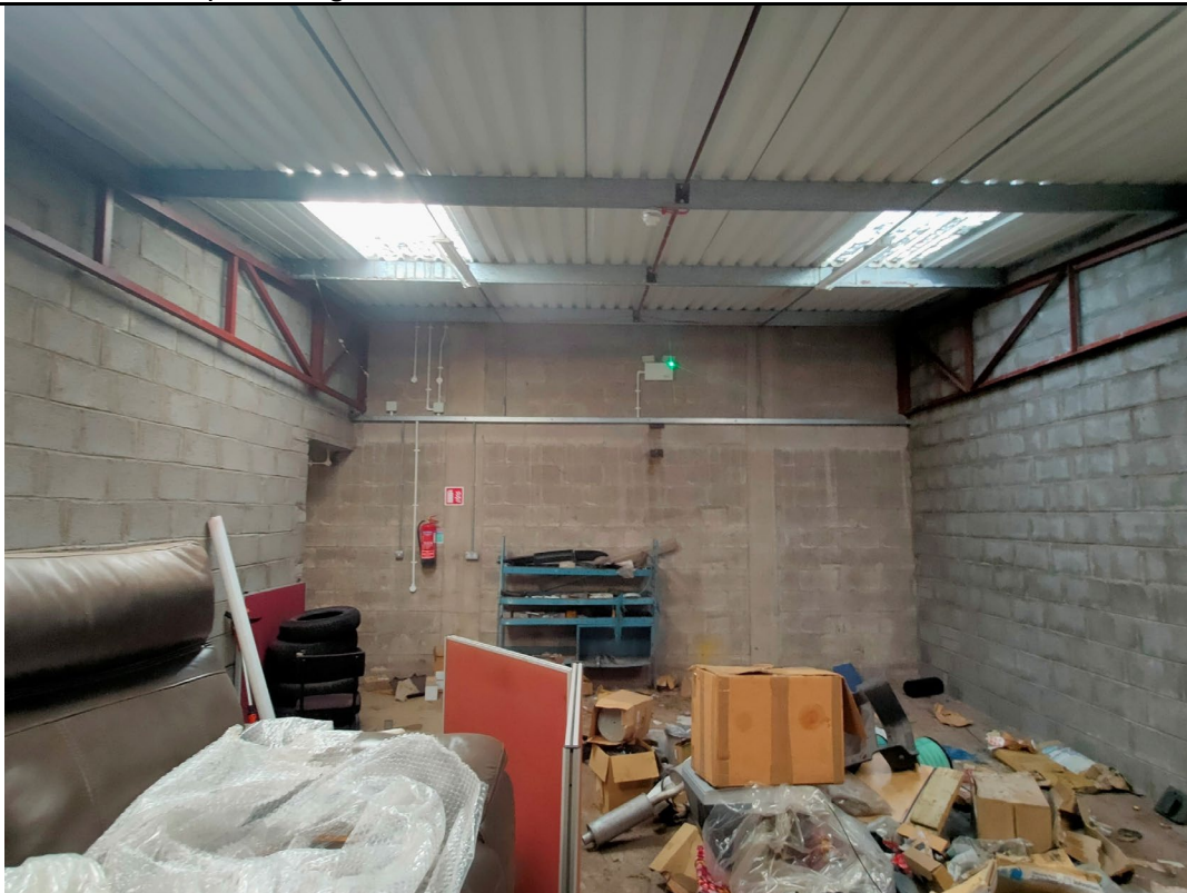
Image 26: View of store room located to north side of main workshop area, block walls, steel framed roof with corrugated aluminium sheeting.
