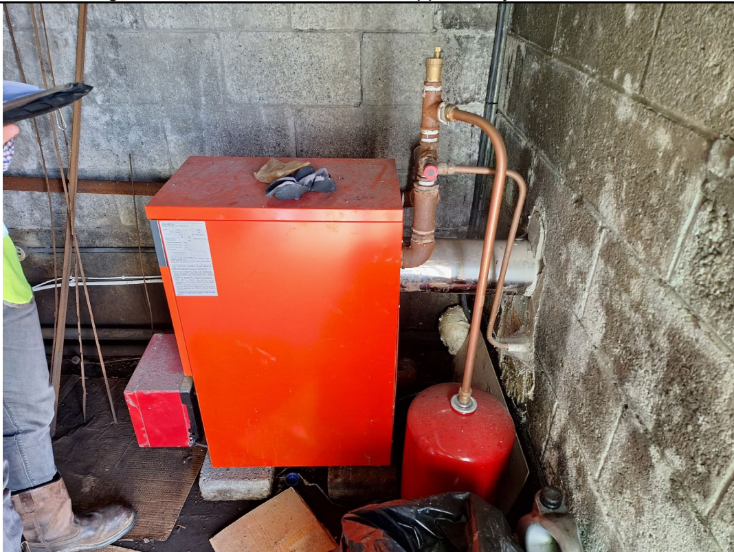
Image 28: View of oil-fired boiler in separate boiler room located at northeast of main workshop.
