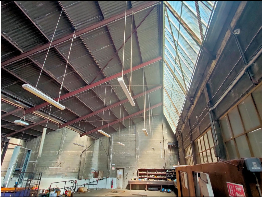
Image 21: View of interior of workshop building, facing north. Offices visible on right. Previous machining work area visible in centre.
