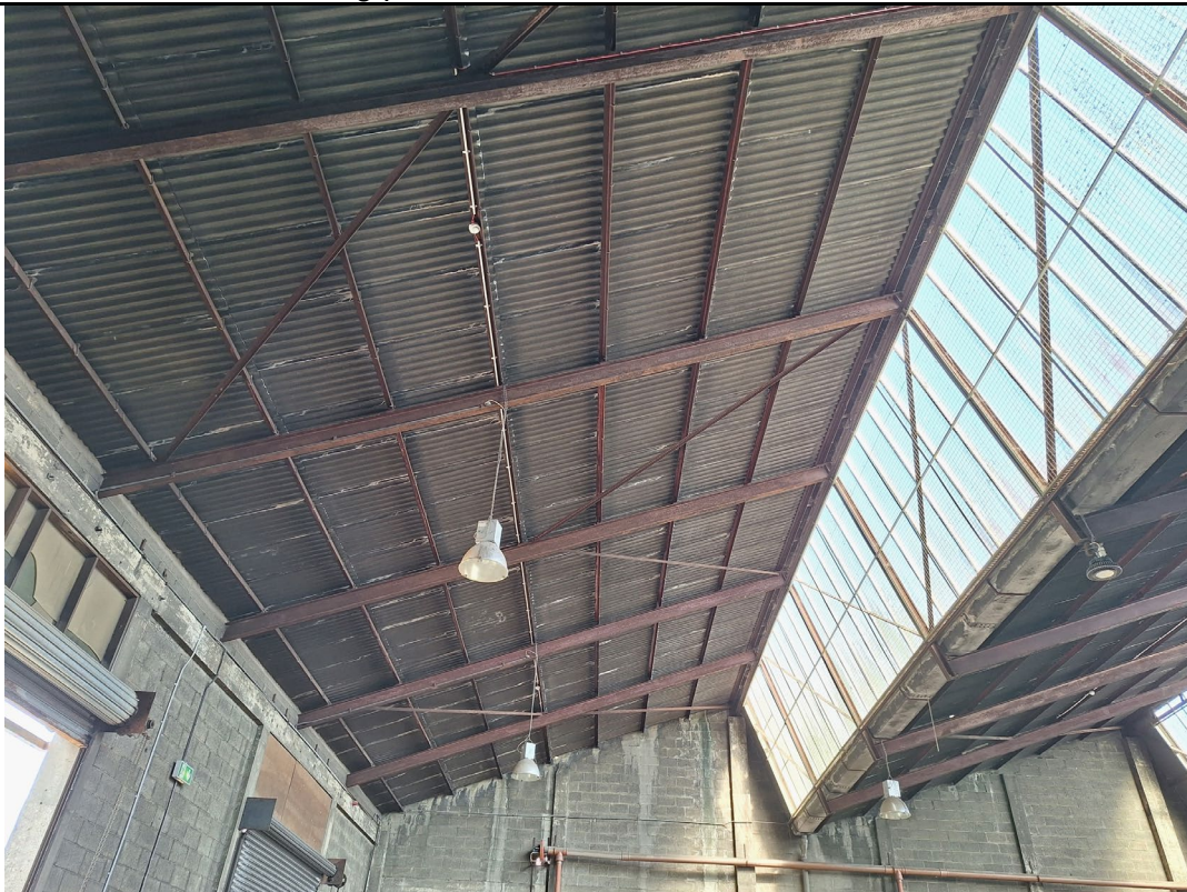
Image 36: View of roof of workshop building, from western entrance, facing north. Roof construction consists of steel beams supported on concrete columns.
