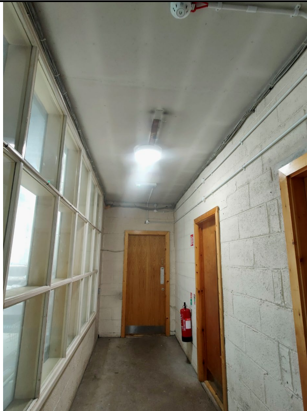
Image 33: View of interior corridor between workshop (left side) and Kildare County Council offices (right side). Polished concrete flooring, painted block walls, glass partition.
