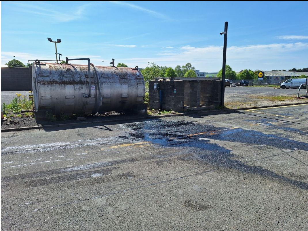
Image 13: View of green diesel AST and concrete block tank plinth south of workshop, facing south. 1 No. 4,500-litre approx. AST (diesel) removed from plinth during audit.
