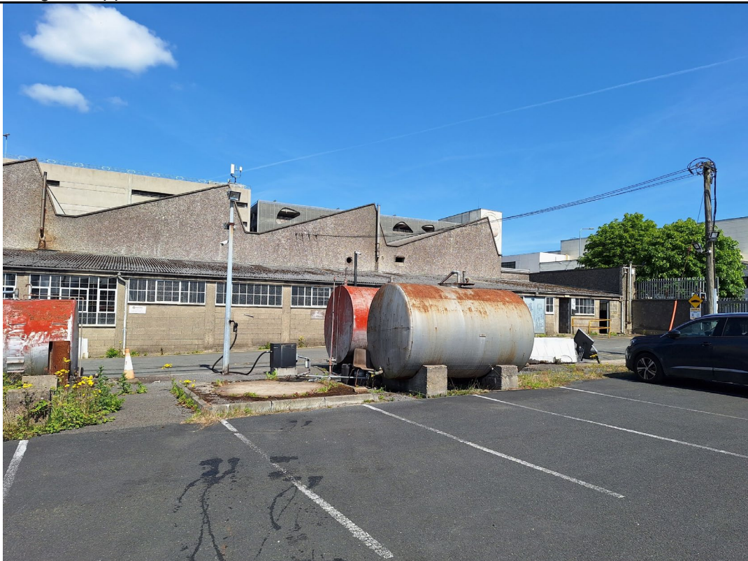
Image 10: View of southeast of workshop building with 3 No. aboveground storage tanks and fuel pump visible. Tanks each approx. 5,000-litre, 2 No. diesel (right), 1 No. green diesel.
