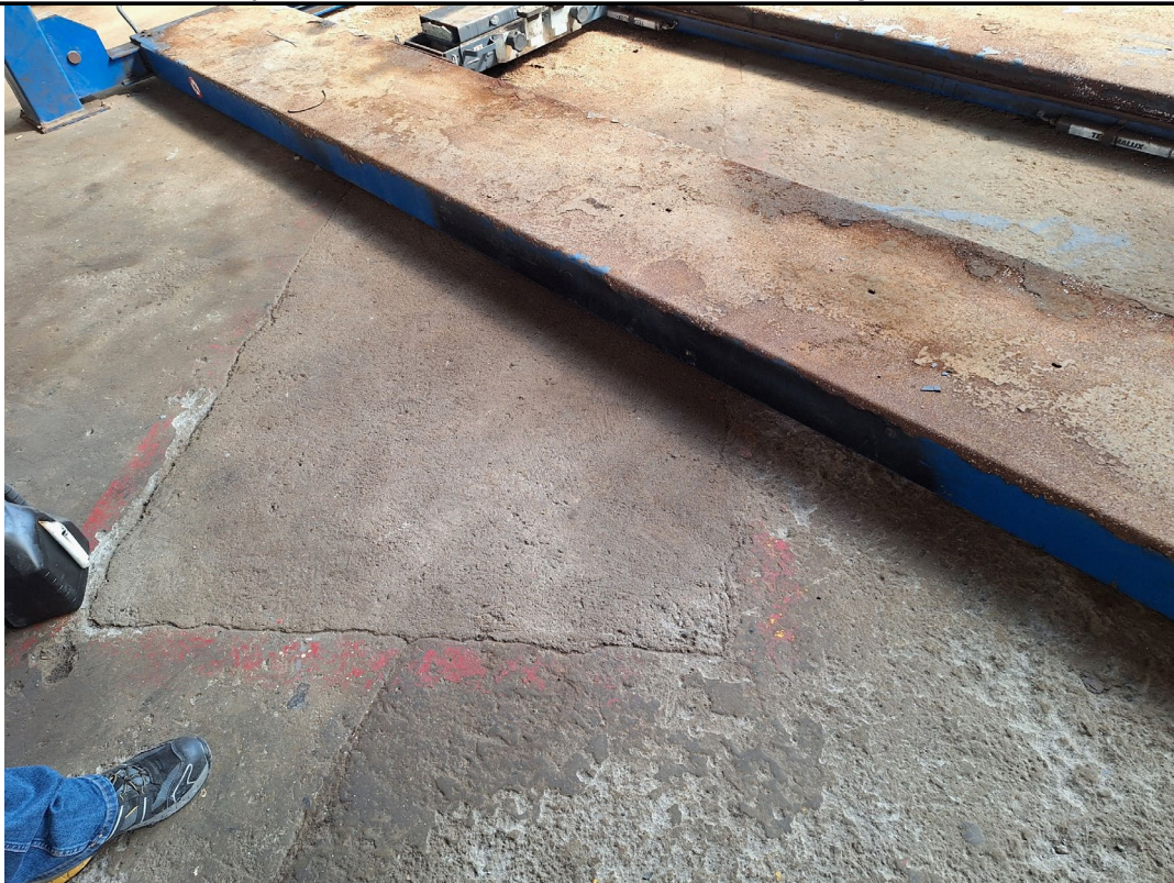
Image 24: View of concrete scar at location of infilled former inspection pit in workshop. 3 No. infilled inspection pits are located within workshop.
