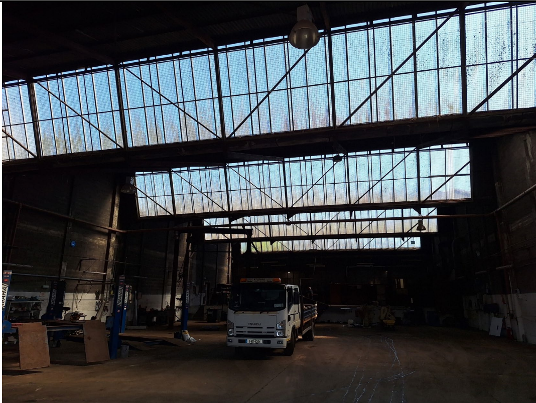
Image 35: View of main workshop, from western side, facing northeast. Hydraulic lifts visible on left, clear roofing panels and steel cross-beams also visible.
