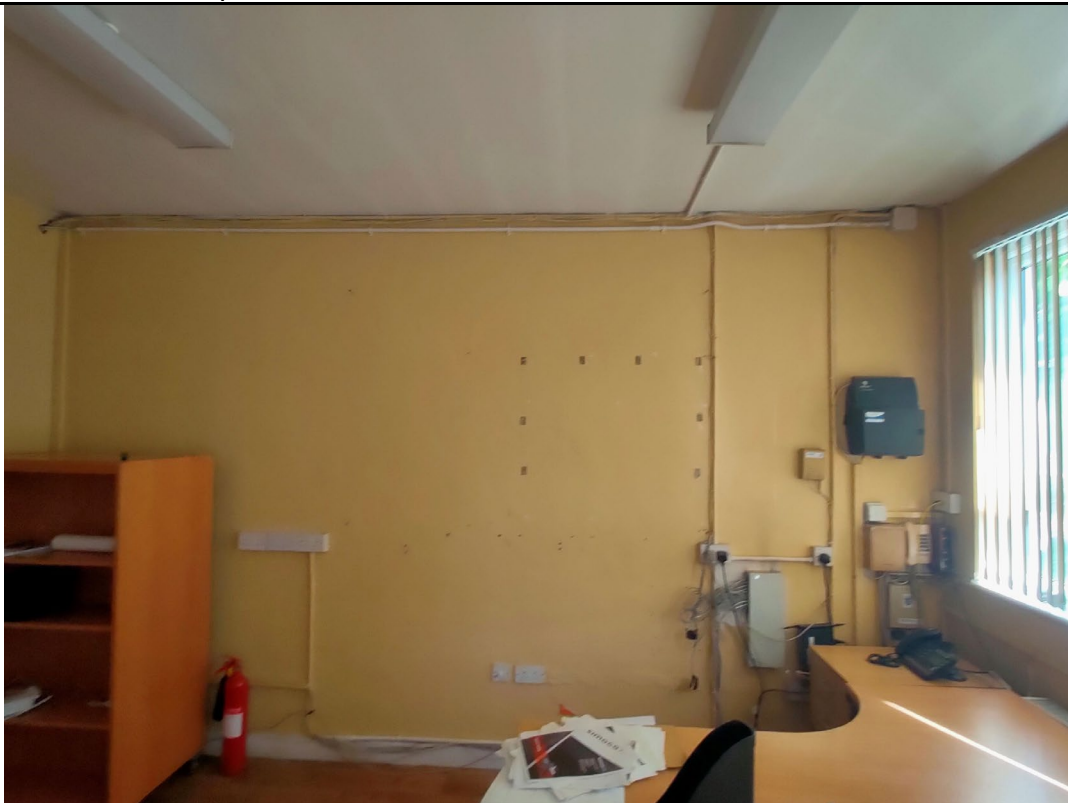
Image 30: View of typical office space on eastern side of main building. Laminate wood flooring, plastered block walls and ceiling, fluorescent lighting throughout.
