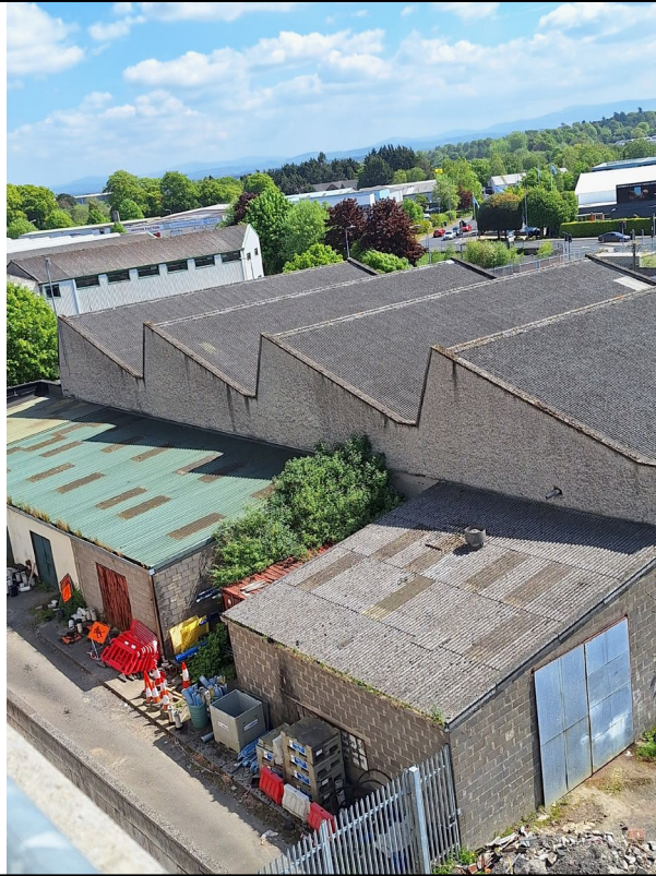
Image 3: View of main workshop building at northeast of site, from northern boundary, facing southeast. External Water Dept. storage yard visible in foreground.
