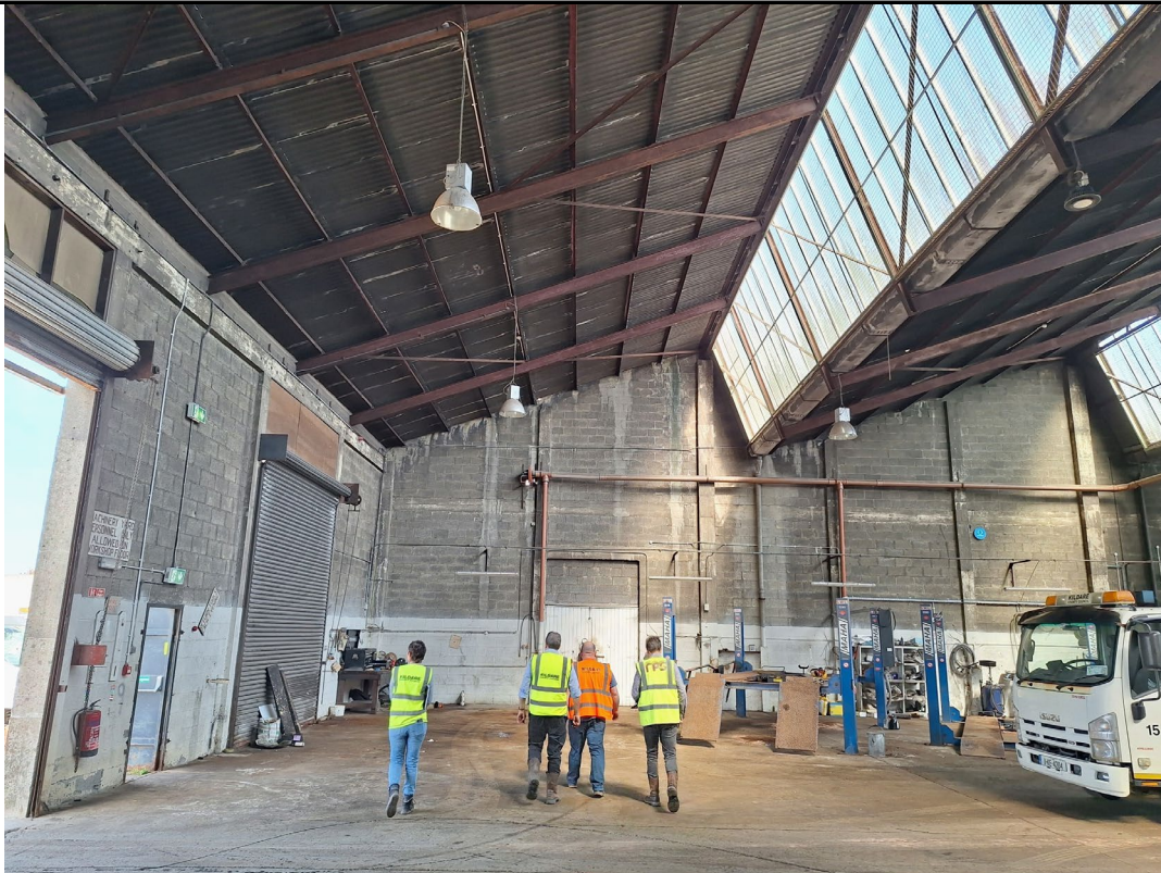
Image 23: View of workshop interior, eastern side, facing north. Roller shutter doors visible on left, 2 No. hydraulic vehicle inspection lifts visible on right, concrete floor
