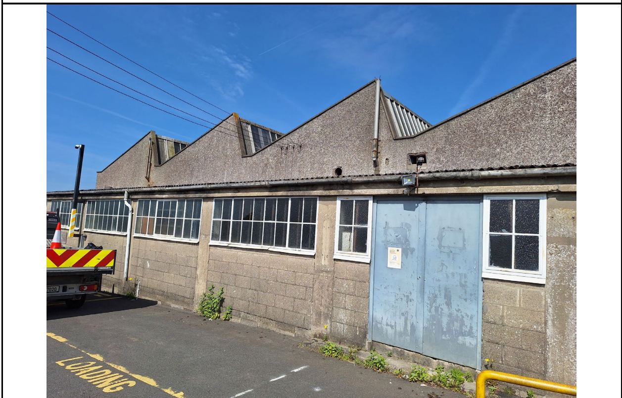
Image 8: View of southeast of workshop building, from entrance road, facing northwest. Concrete block wall construction and sawtooth corrugated roofing visible.
