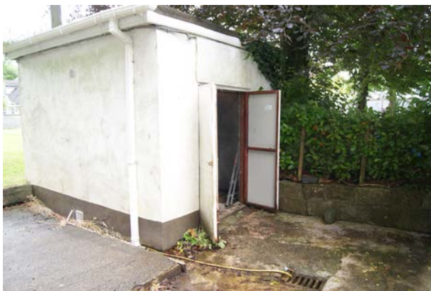
Photo 1 – Pump House at Ballindoolin GWS (note: drain cover in foreground represents position of old, shallow, local authority well)
