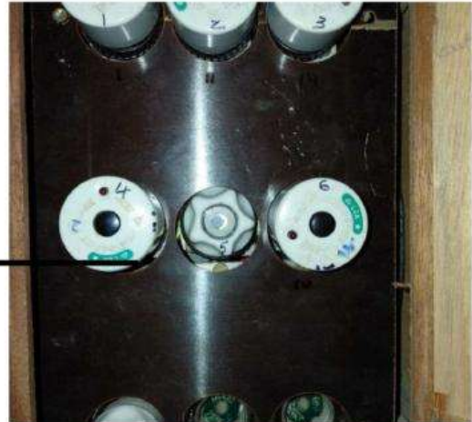
SDB CERAMIC SCREW-IN FUSES
