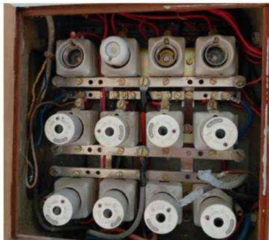
SDB CERAMIC SCREW-IN FUSES
