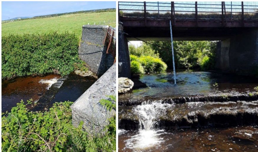
Figure 2 Killeen Bridge Apron Barrier
