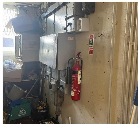
MAIN DISTRIBUTION BOARD ARRANGEMENT
