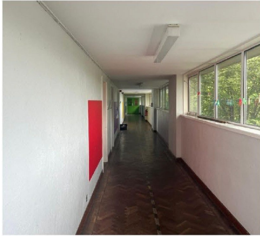
CORRIDOR - NO EMERGENCY LIGHTING/ FDAS COVERAGE
