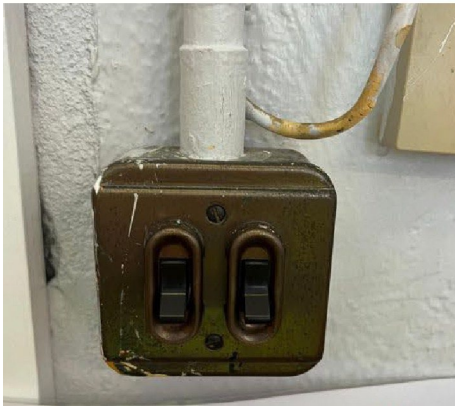
Fire Exit Room 31
