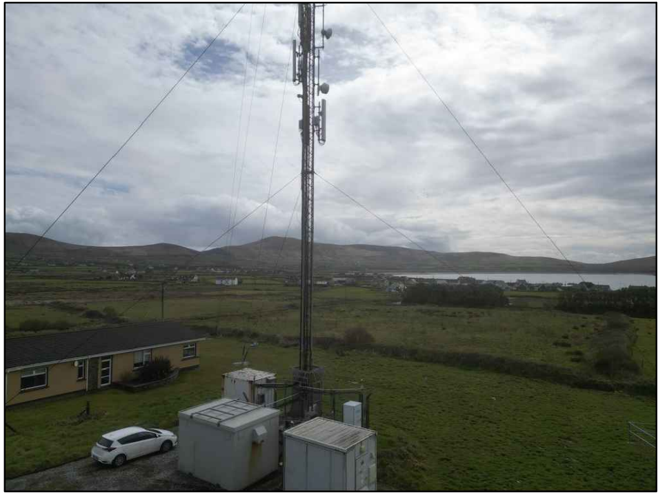
Fig 1. Existing Mast Elevation Photograph
