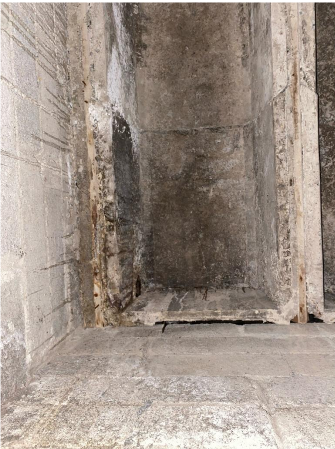
Figure 5: water ingress from failure of roofing felt is dripping down and saturating ceiling underneath. Photo taken from removed area of ceiling looking up toward underside of concrete roof. Note the staining and mould from condensation due to lack of insulation in the roof
