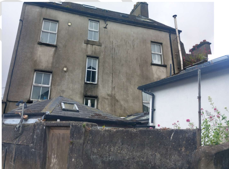
Figure 1-3 View of the Rear of 13 Market Street
