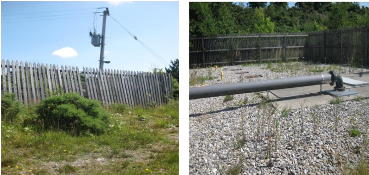
Figure 35: The dilapidated timber fencing surrounding the Kilmovee Urlaur water treatment plant.
