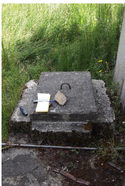
Photo 5: External pump sump access
