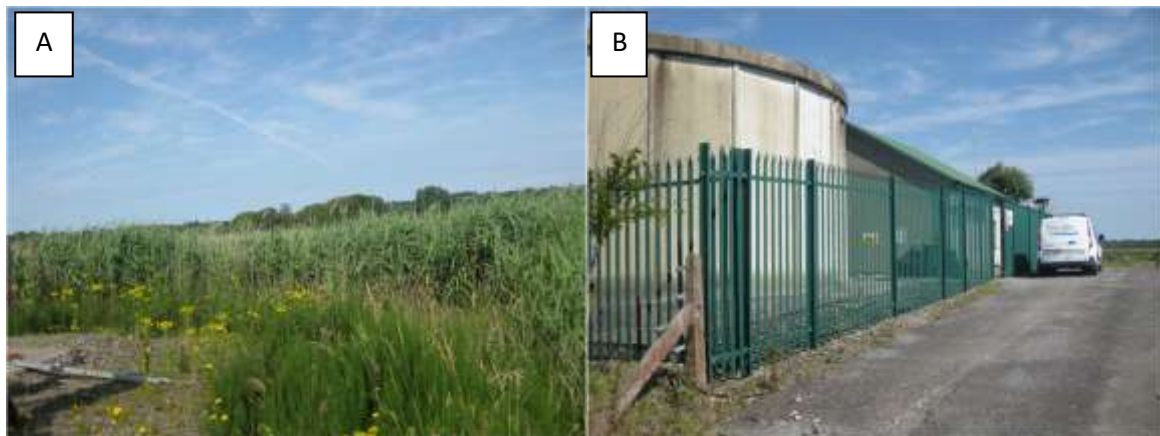
Figure 1: Site Location: A) Lough Caheer is surrounded by reeds, with raw water storage tank to the left of the photo. B) Brackloon Spaddagh GWS water treatment plant and storage reservoir.
