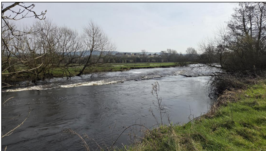
Plate 1 Ballyragget Weir from upstream right bank during high flow conditions
