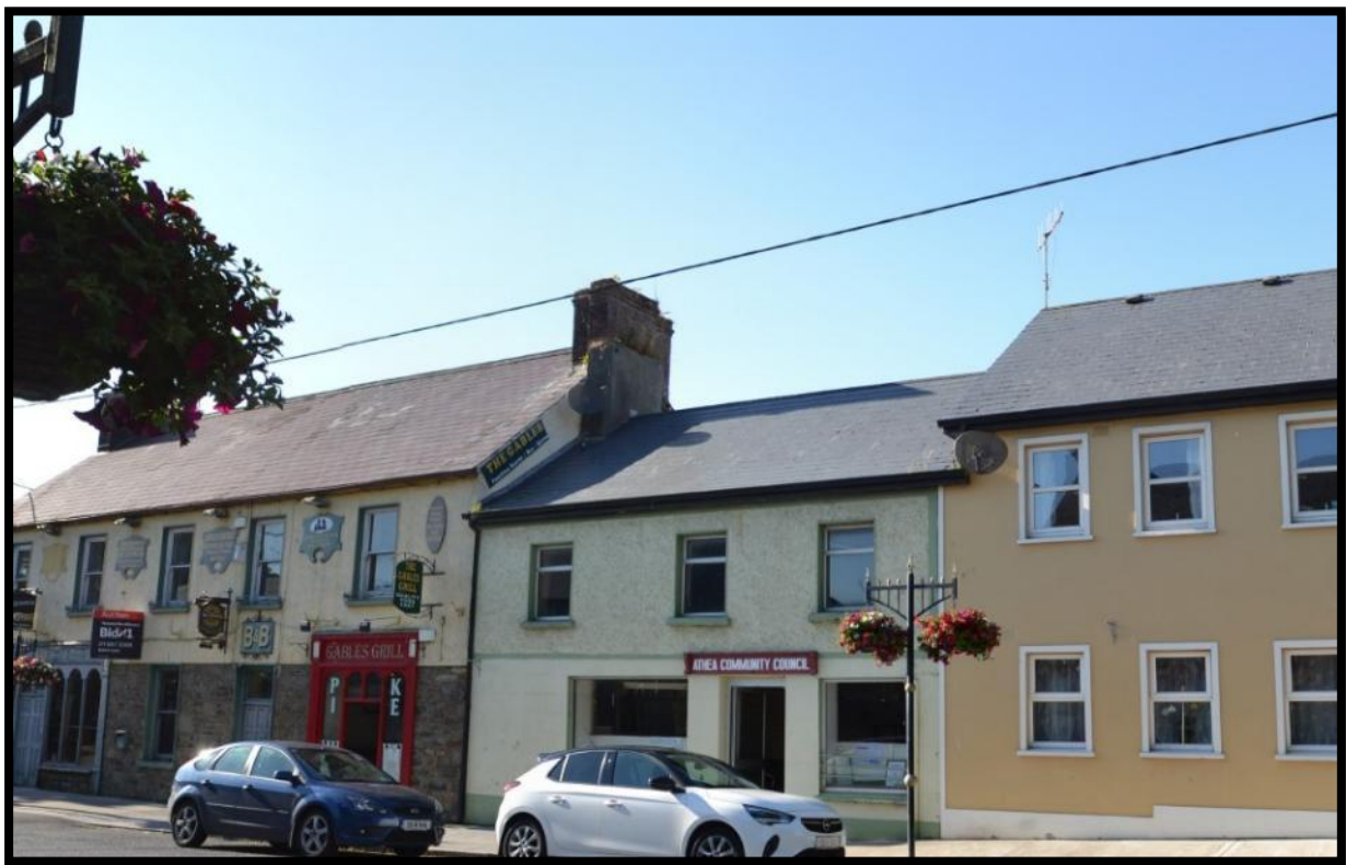
Fig. 1: View of Athea Community Council Building, Colbert Street, Athea, Co. Limerick.
