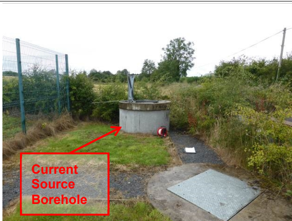
Photo 4: View WSW over Current Source Borehole
