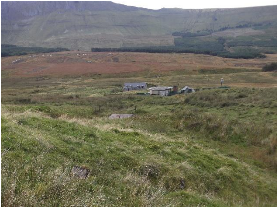
Photo 6. Collection Tank for flow from Spring 1 in mid ground. Treatment plant and reservoir in background.
