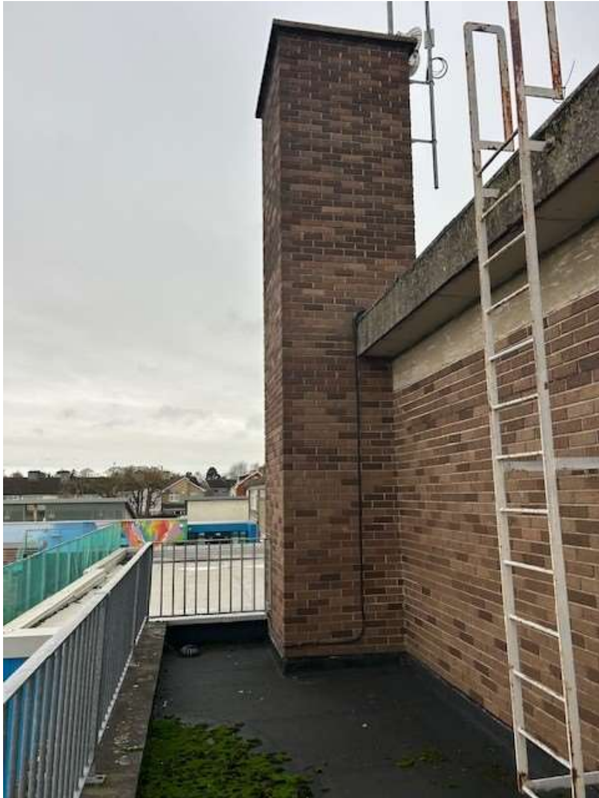
Exterior view of the balcony outside Classroom 11, from balcony level, with existing roof finishes and roof access ladder
