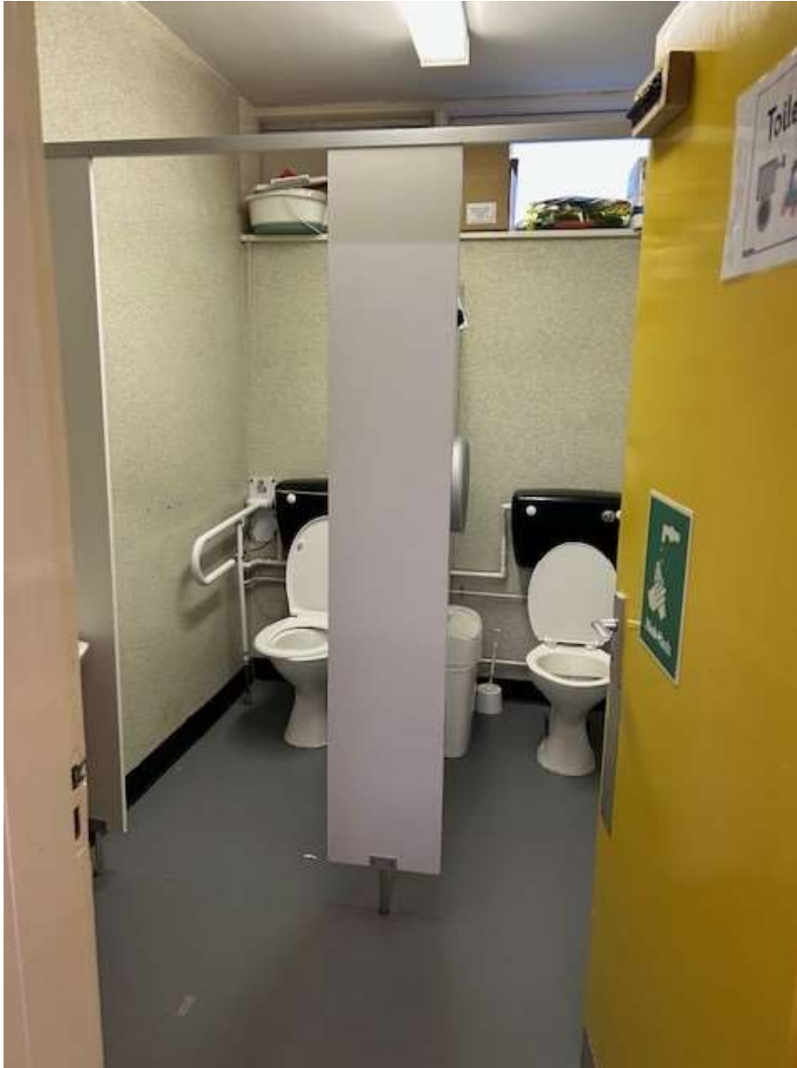
Classroom 3 – Exterior view existing toilets
