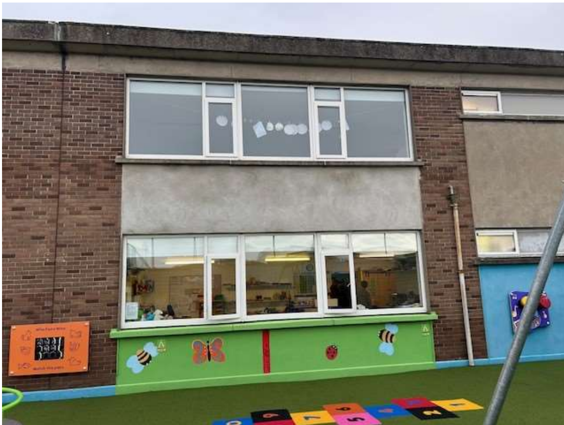
Classroom 3 – Exterior view of wall for new external door
