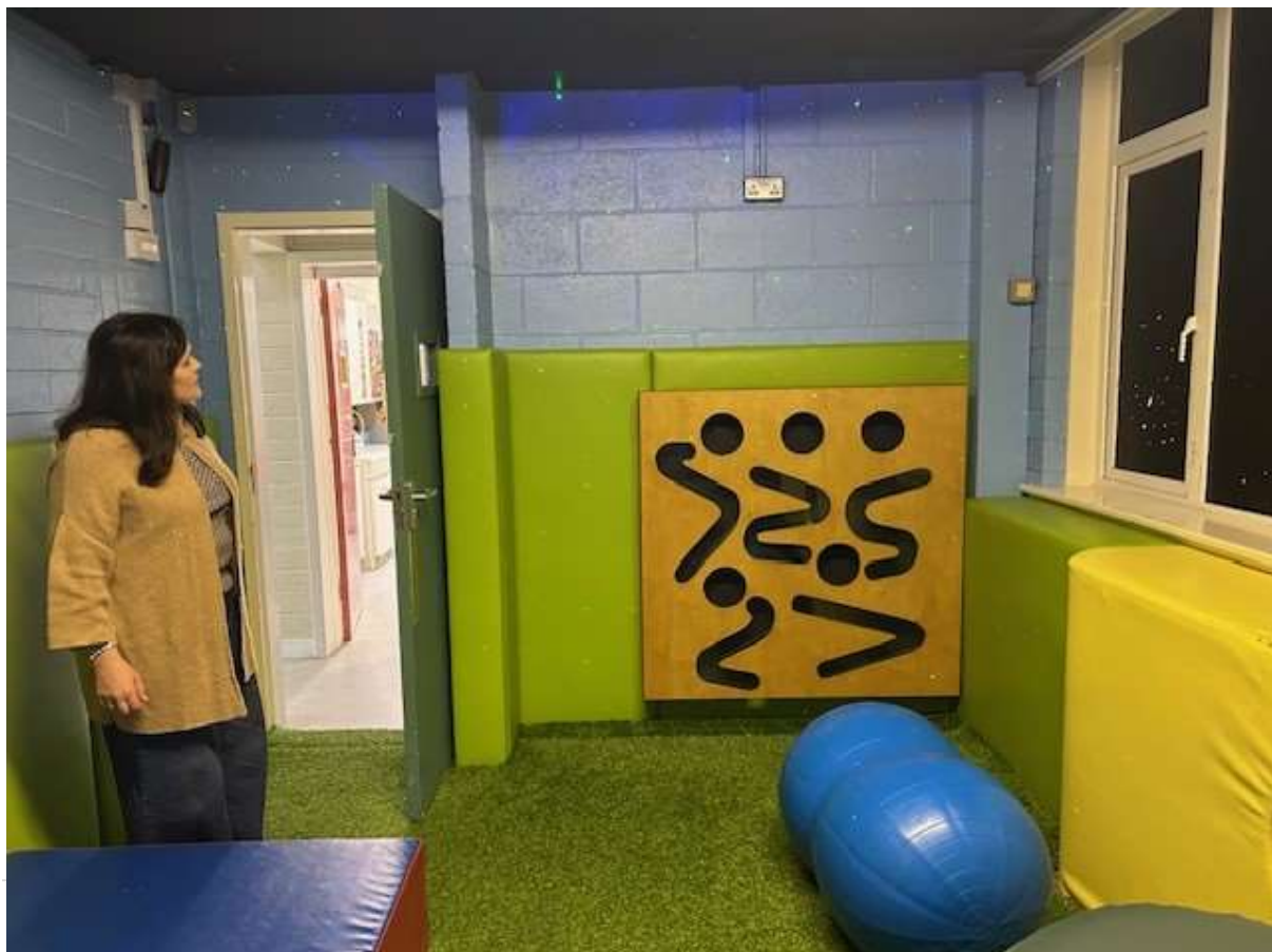
Snoezelen – Interior view of room with no ventilation.
