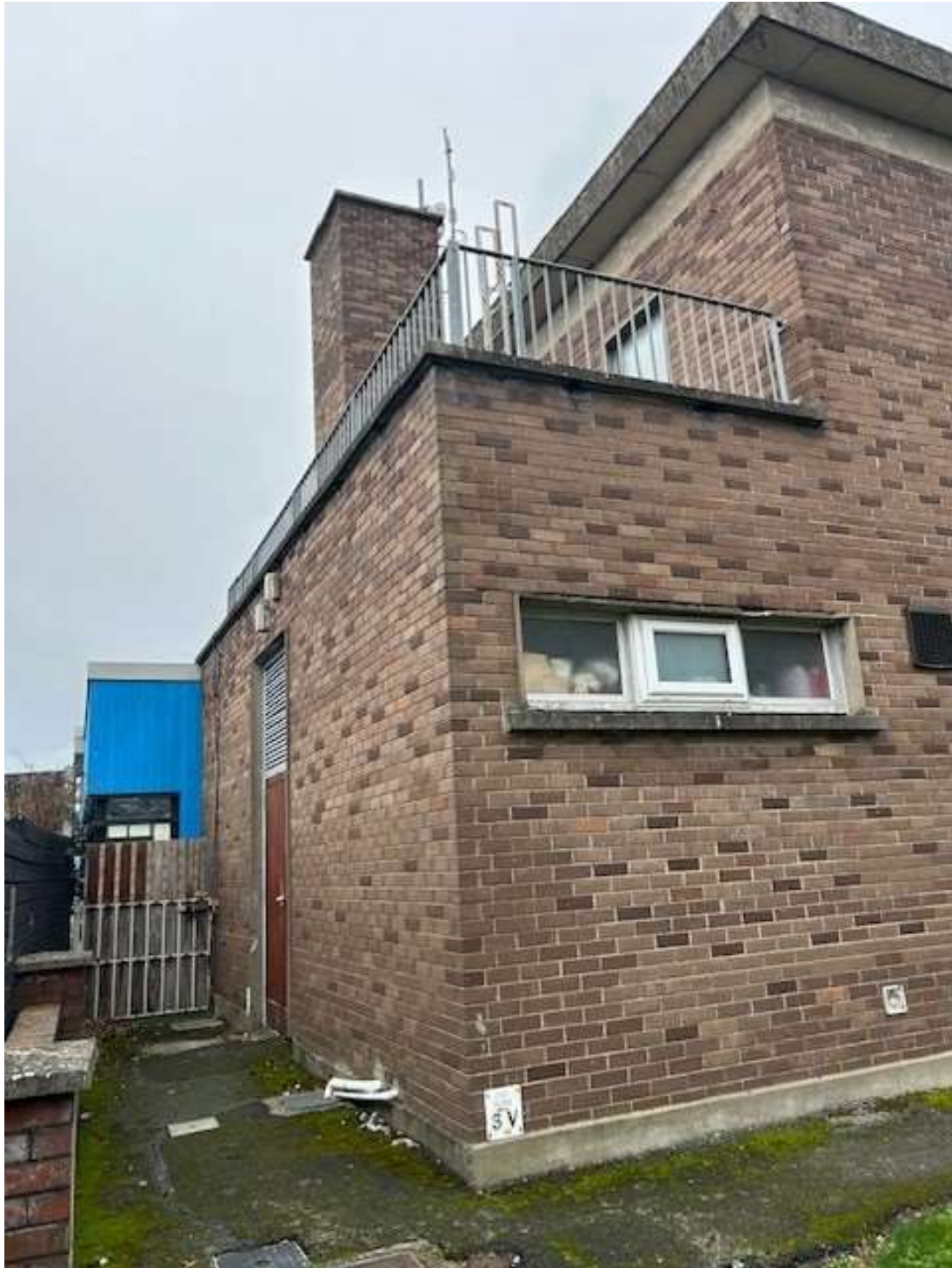
Exterior view of the balcony outside Classroom 11, from ground level, with storeroom window to be blocked up to allow fire escape stairs to pass.
