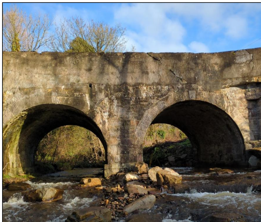
Figure 4 Photo of Cahernahallia Bridge Apron
