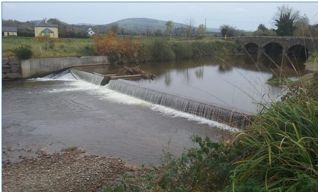
Figure 8 Photo of Blackboy Weir
