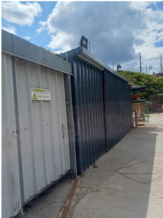
Floodlight at the boat yard
