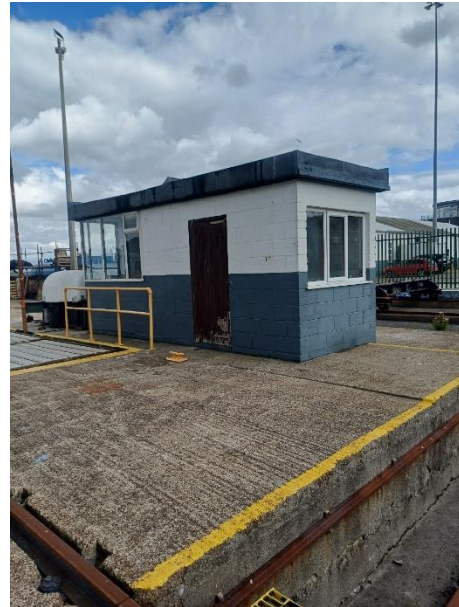
Syncrolift Control Building
