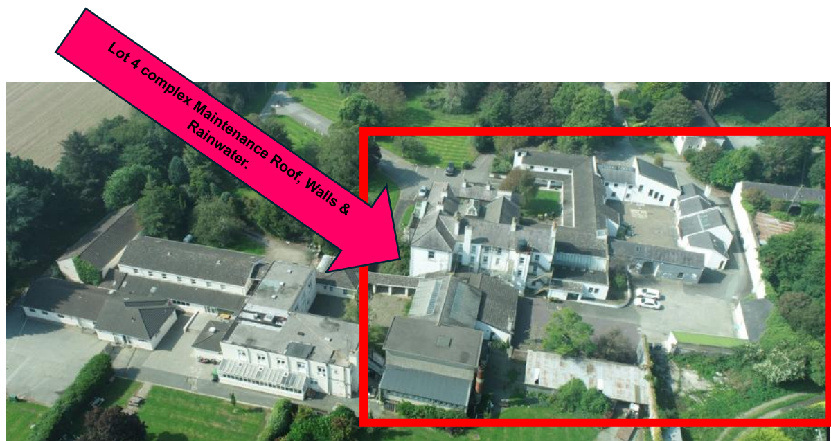
Figure 2 An Grianán Adult Education College Complex Lot 4 Annual Maintenance Contract for Complete Complex Roof, Walls & Rainwater.
