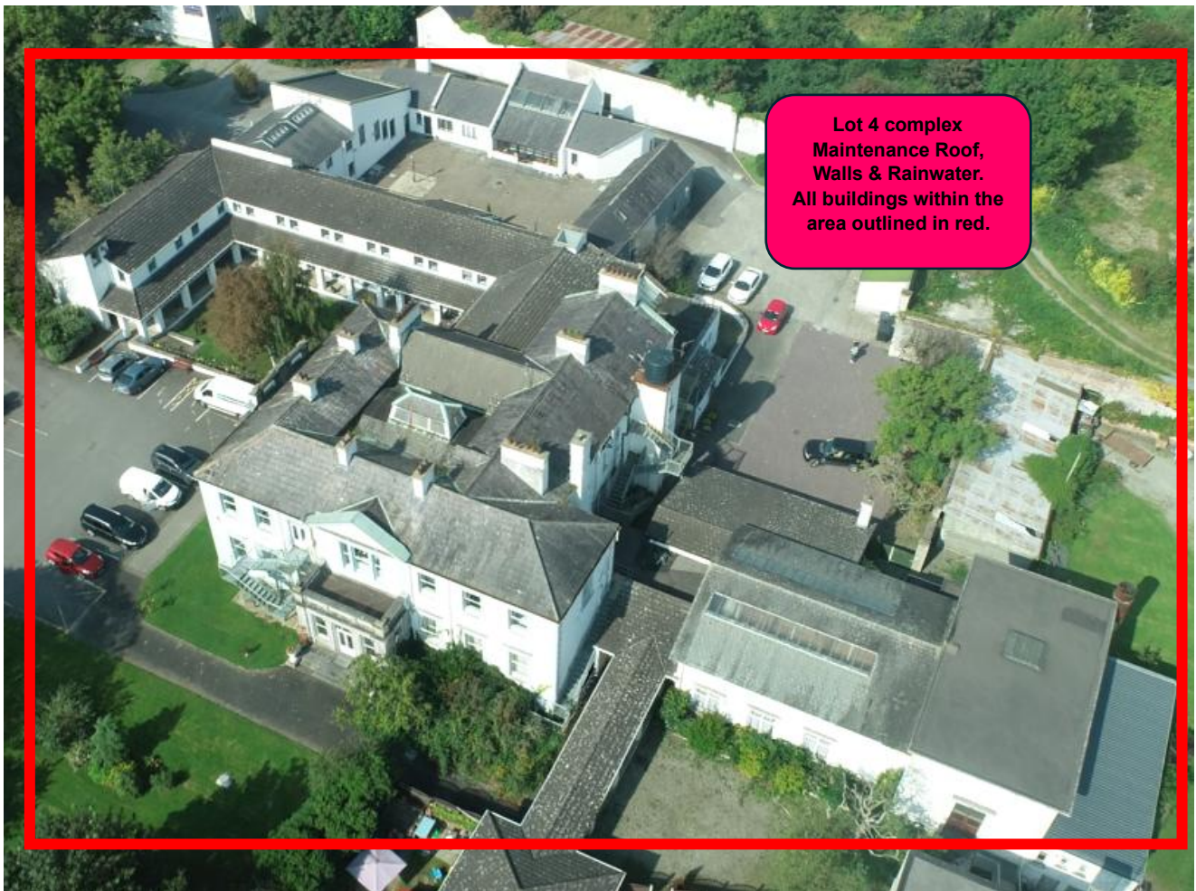
Figure 9 LOT-4 Annual Maintenance Contract for Complete Complex Roof, Walls & Rainwater.
