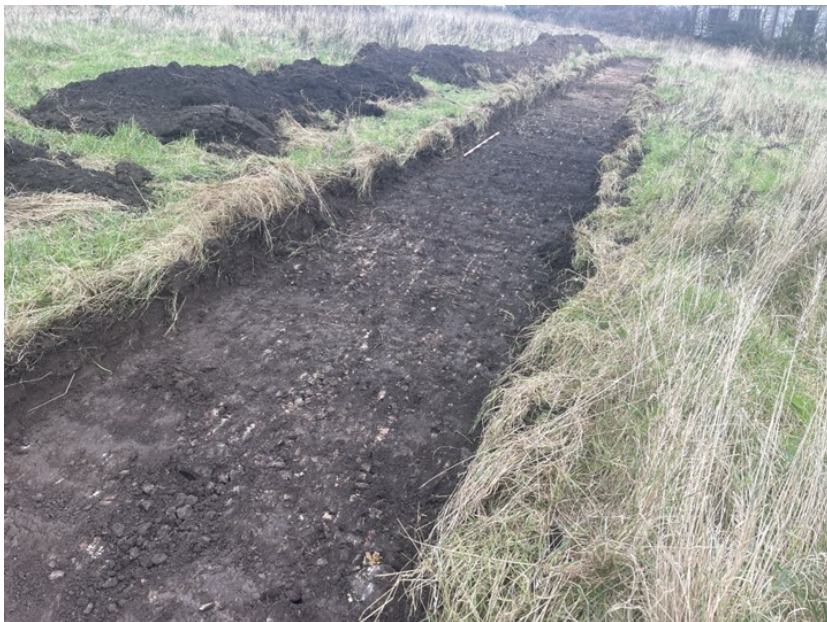
Plate 13: Trench 2 C4 facing North
