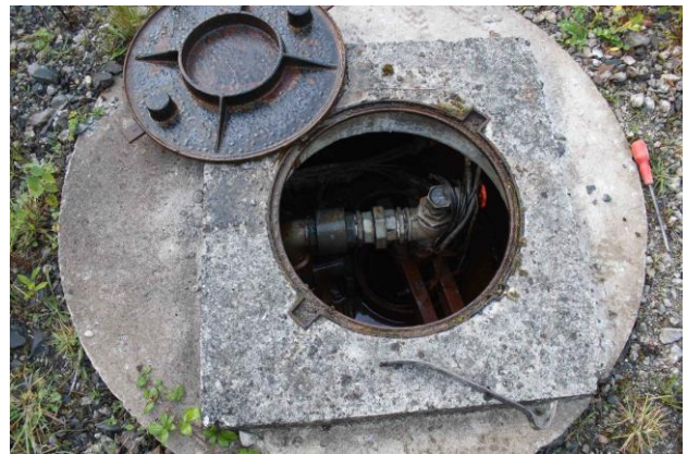
Photo 2: Borehole cover (PW1)
