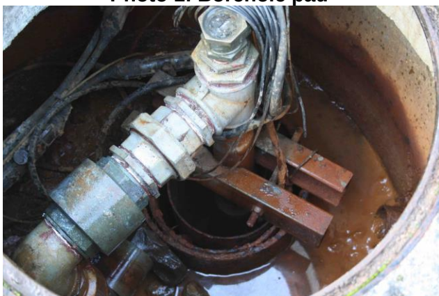
Photo 3: Wellhead arrangement
