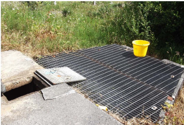
Photo 3: GWS collection box, with overflow weir (under yellow bucket) adjacent to LA sump (with open access point)
