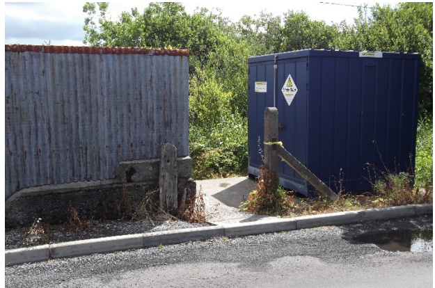
Photo 2: LA chemical storage shed (right) and roadside kerb installed by GWS
