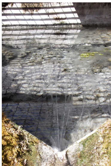
Photo 4: Looking into gravel base of collection box, through v-notch overflow weir
