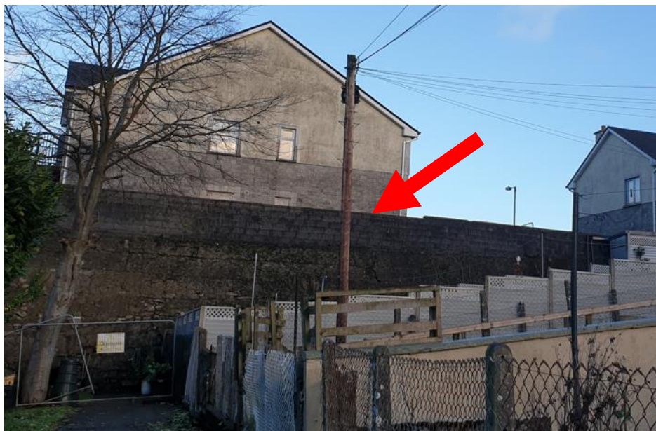
Photograph 2 West face of structure – Note block built wall over original structure.
