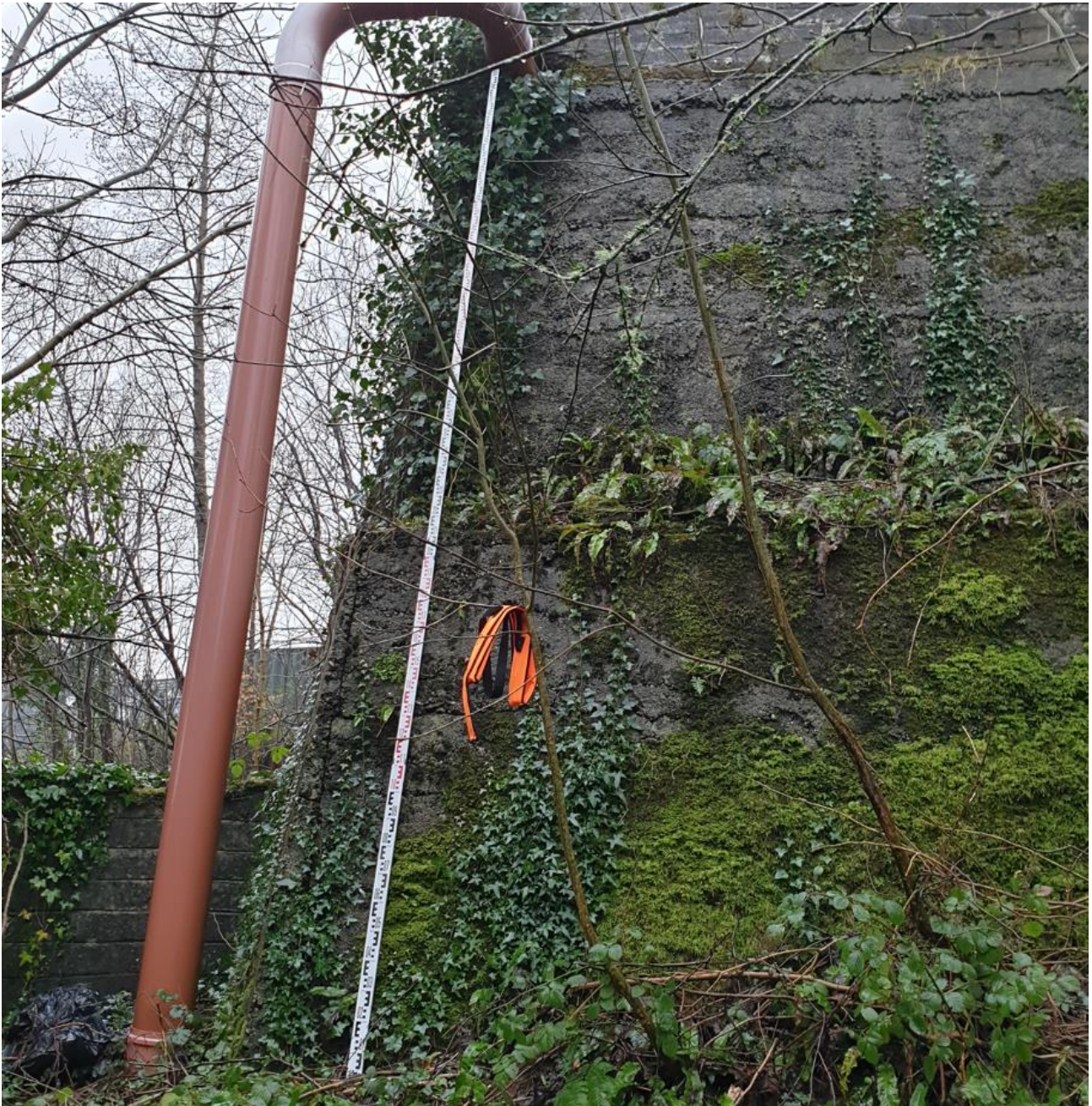
Photograph 12 North Eastern corner of structure – Note 5m measuring staff.
