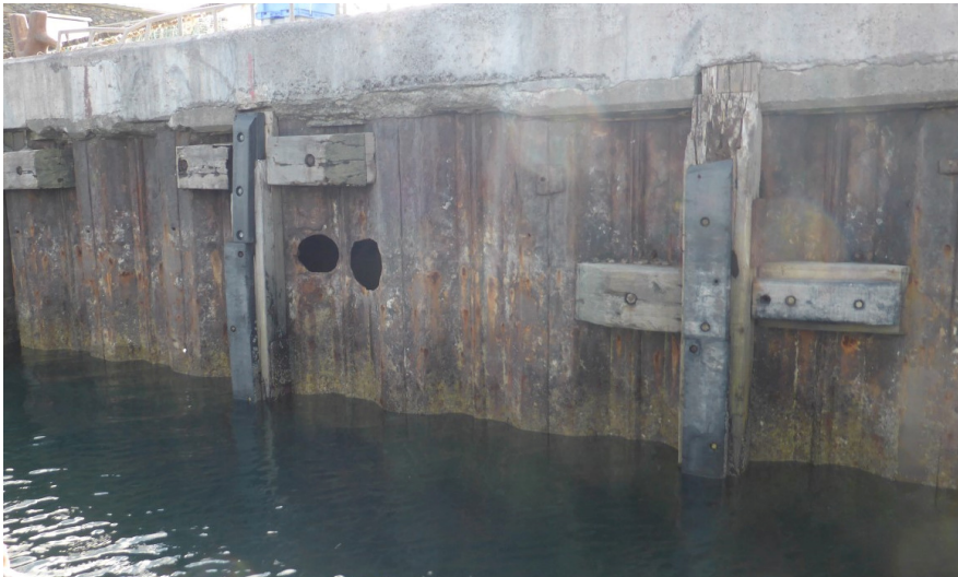
Plate 6 – Holes in sheet piles
