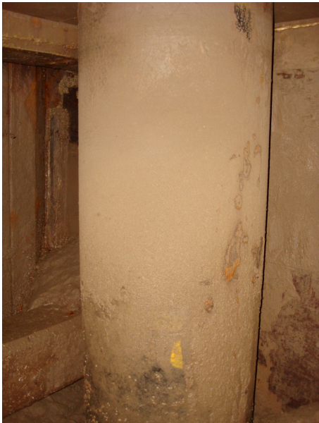
Plate 8 – Typical view on tubular steel bearing pile
