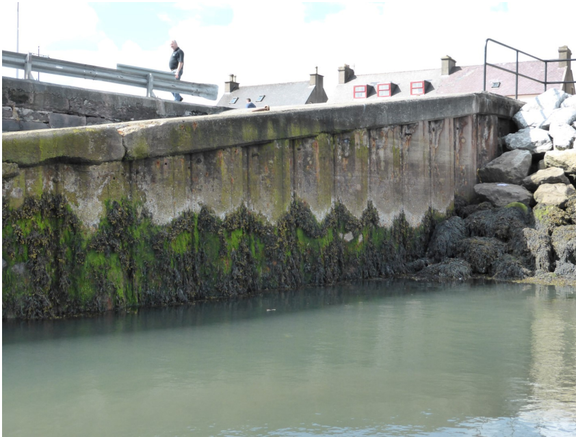
Plate 7 – Typical view on Punt slipway sheet pile wall
