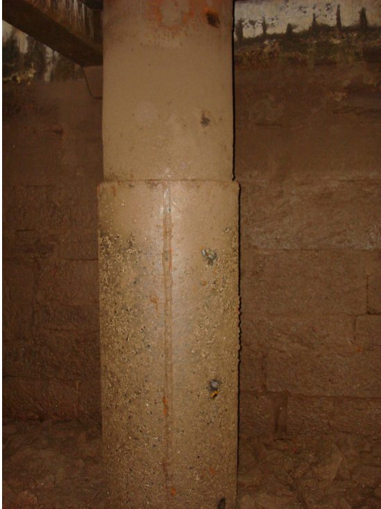
Plate 2 – Tubular steel bearing pile with collar prepared for testing
