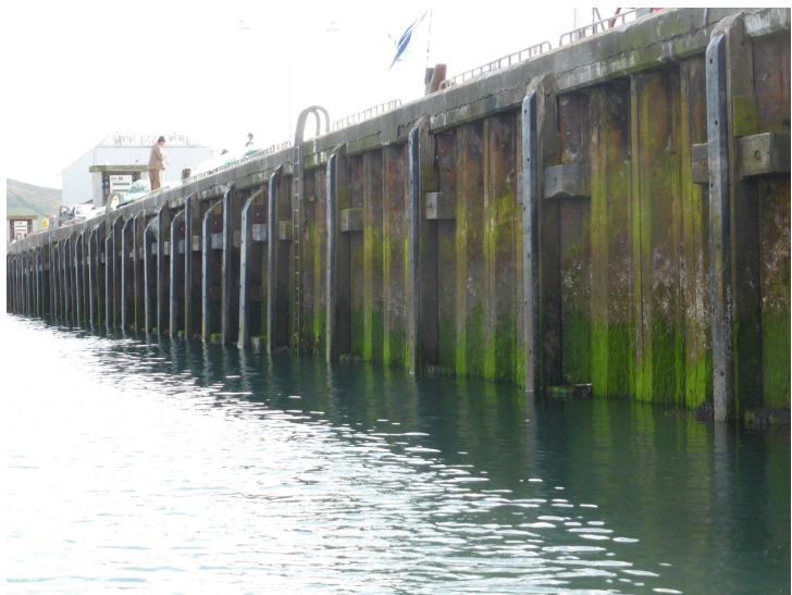
Plate 1 – Typical view of Eastern face sheet pile wall
