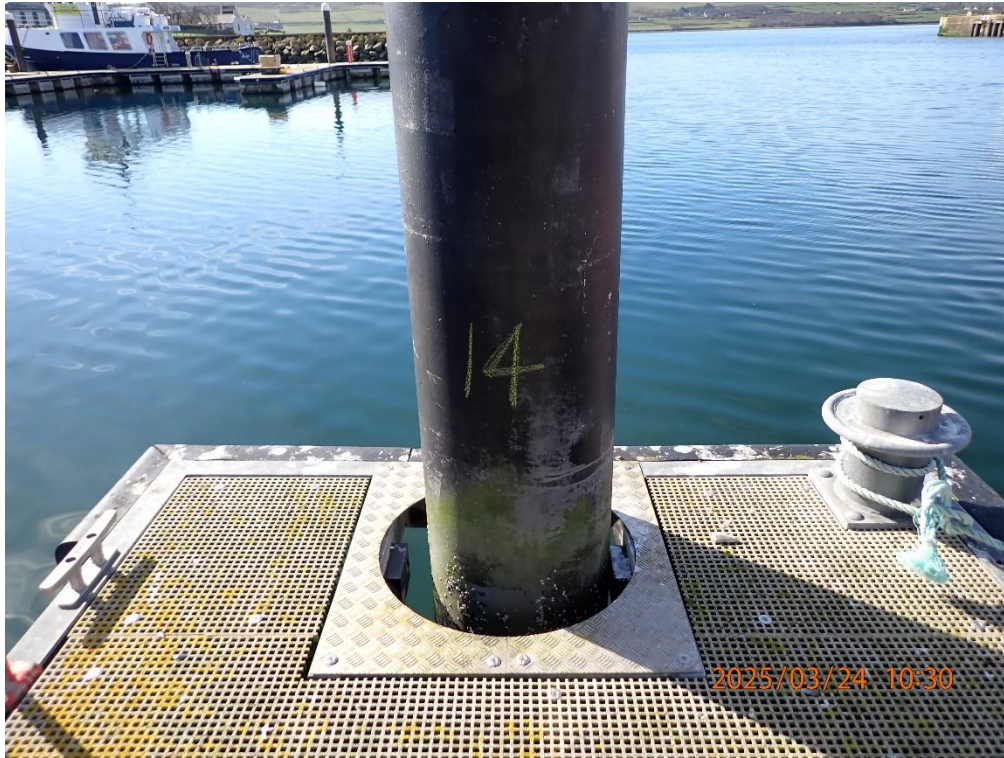
Photograph 7: Typical pile above water
