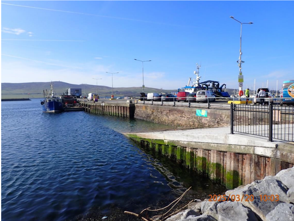
Photograph 1: East face of the Main Pier
