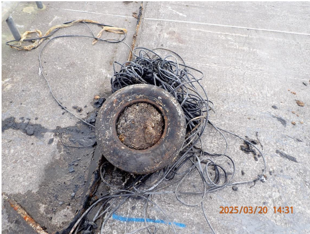
Photograph 27: Debris recovered from the east pier
