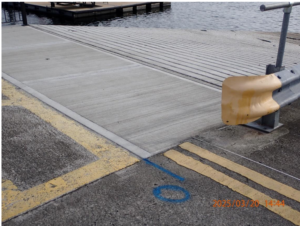
Photograph 8: Ch 0 at the slipway/tarmac interface
