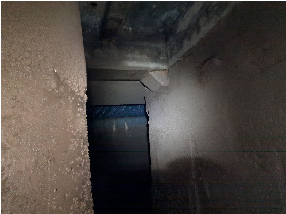
Visual Inspection; Main Pier Supporting Structure, An Daingean Fishery Harbour Centre - March 2026
