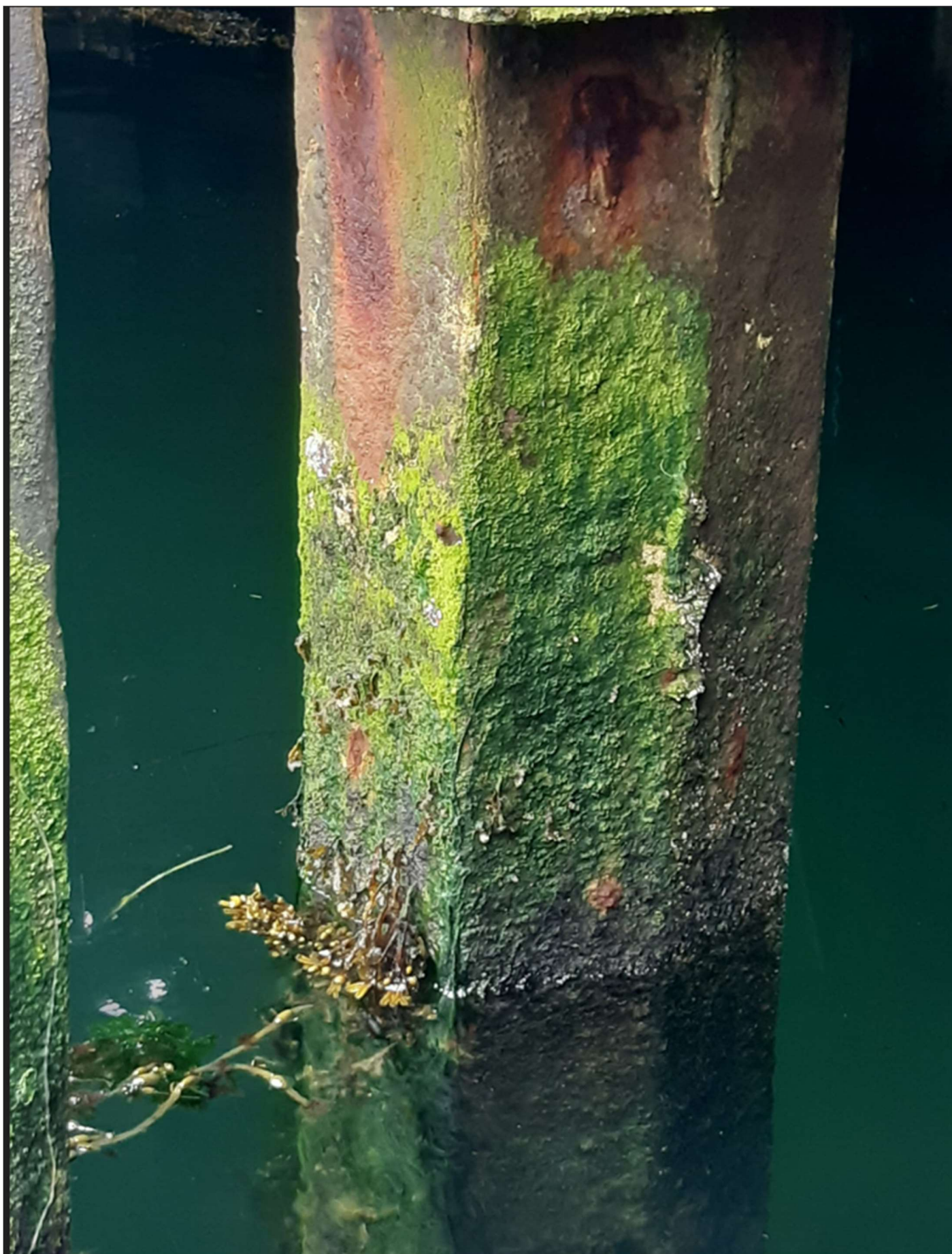
Piles under Main pier
