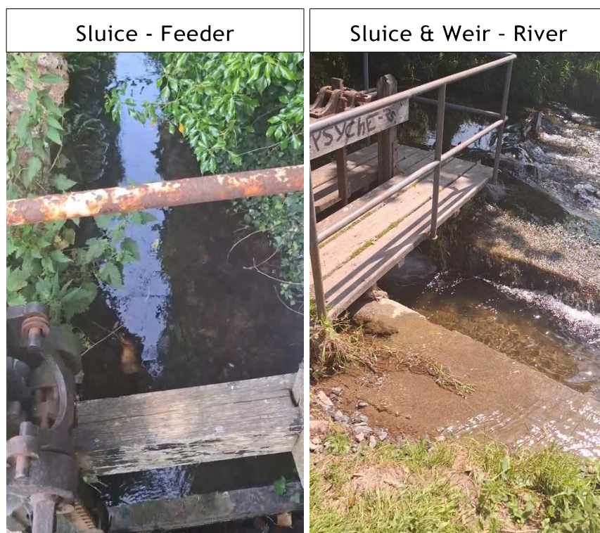
Figure 3-13; Morell Feeder & River Flow controls
