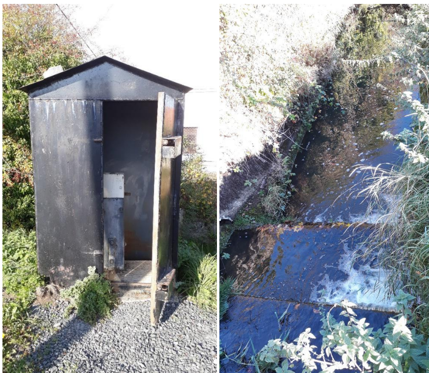
Figure 3-7; Sluice House & Stepped Weir on Rye Water
