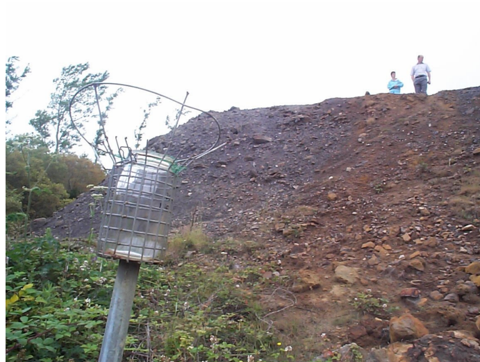
Figure 3.3 Gauge Wa looking towards embankment of TMF
