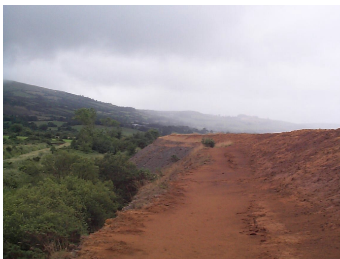
Figure 3.4 Photograph of the east boundary of the TMF looking south
