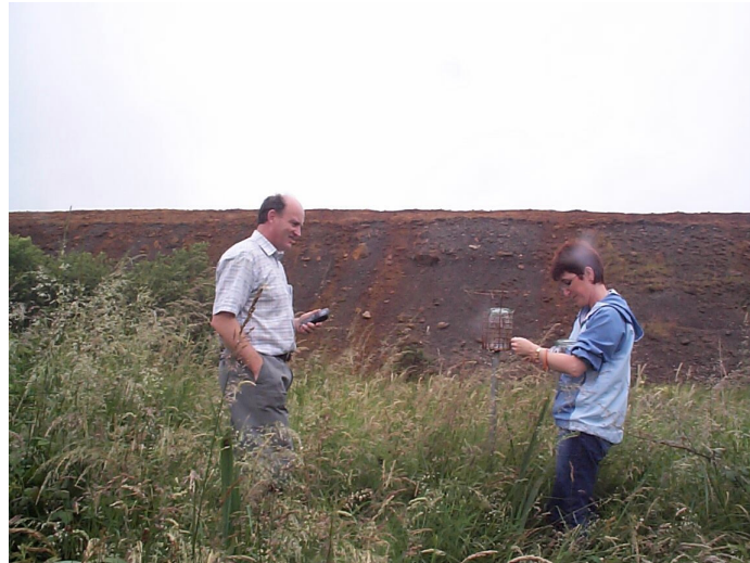
Figure 3.2 Gauge Ea, with view of embankment in background
