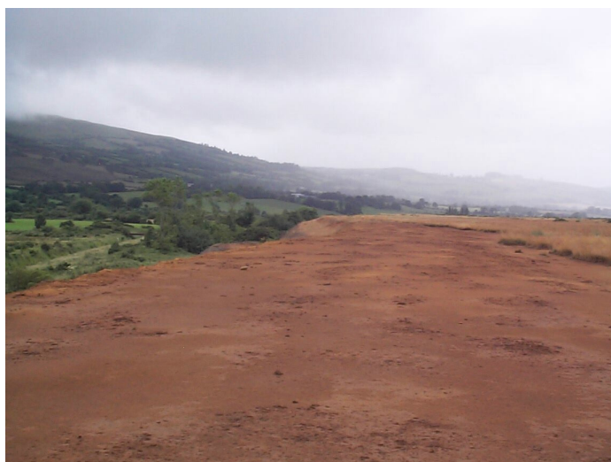
Figure 3.5 Photograph of surface of TMF above East gauge
