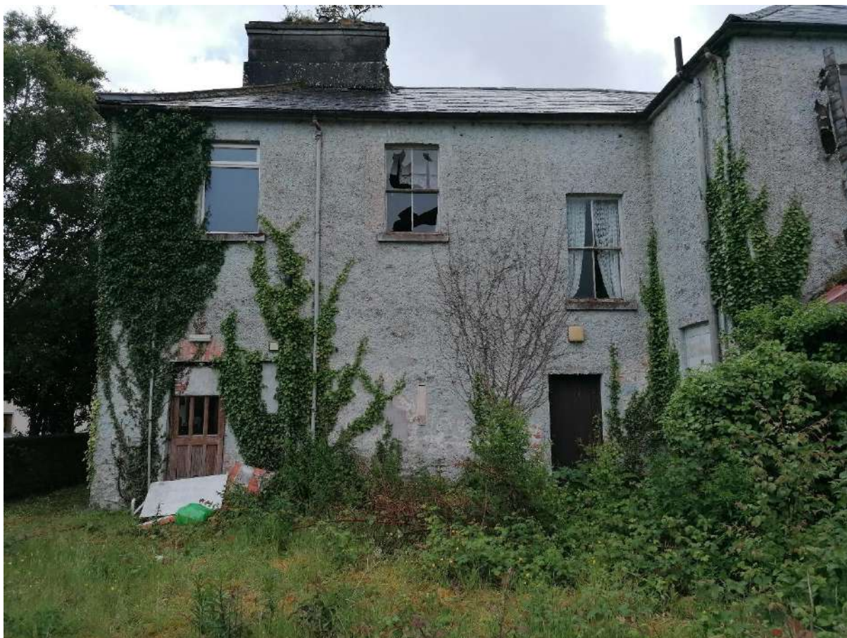
Fig. 3 Rear (North West) elevation
