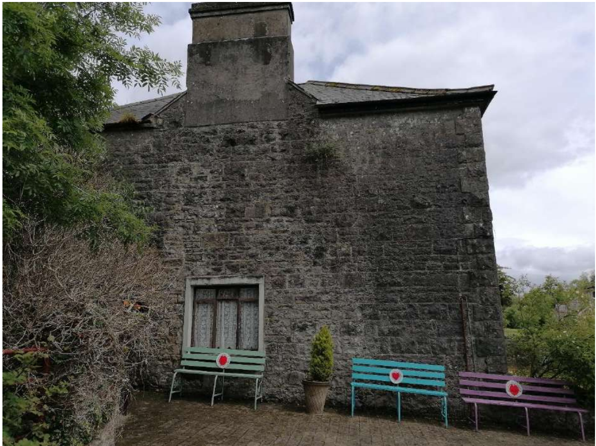
Fig. 2 Side (South West) elevation
