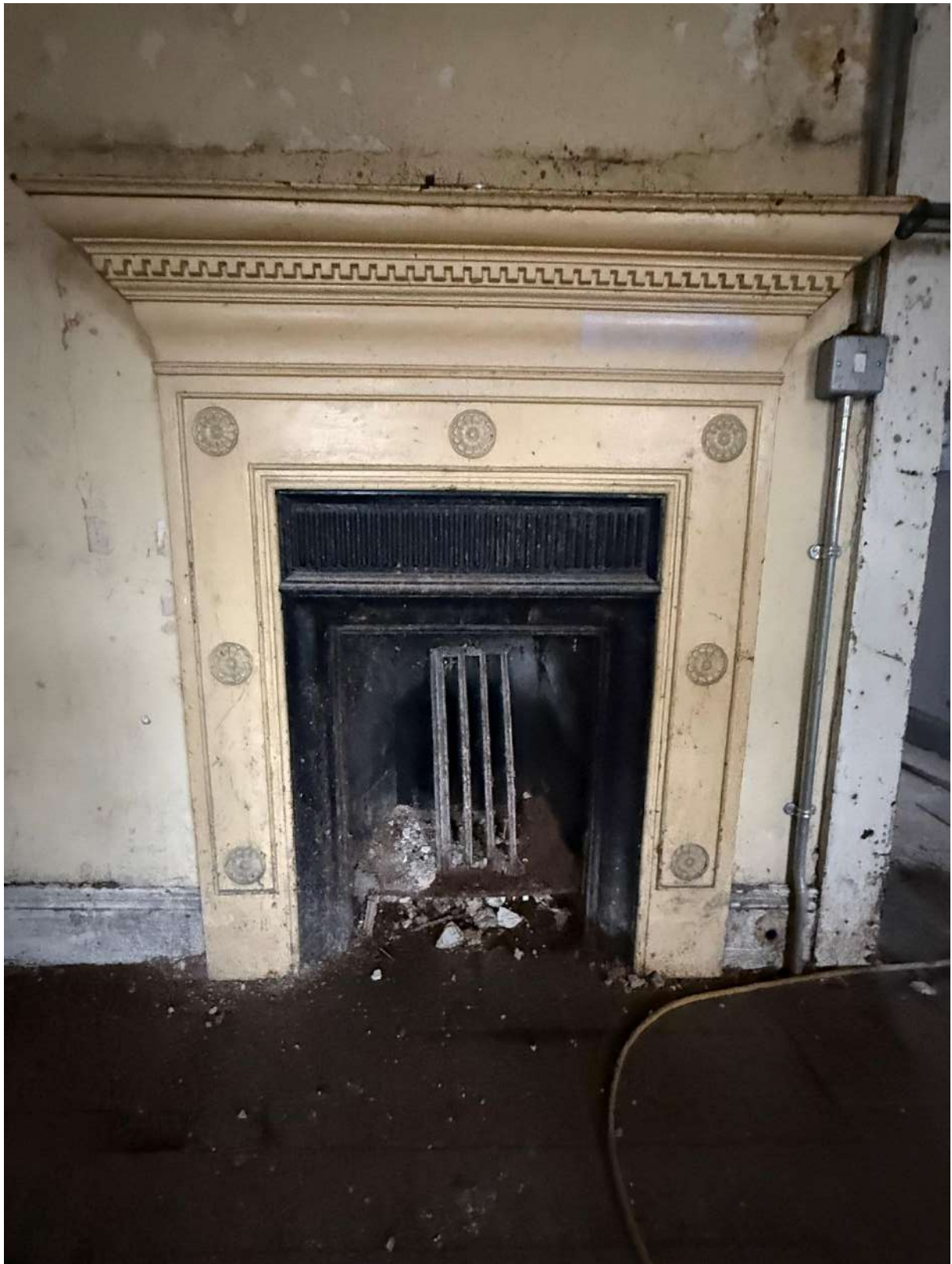
Fig. 14 Original fireplace to Eastern front room at first floor
