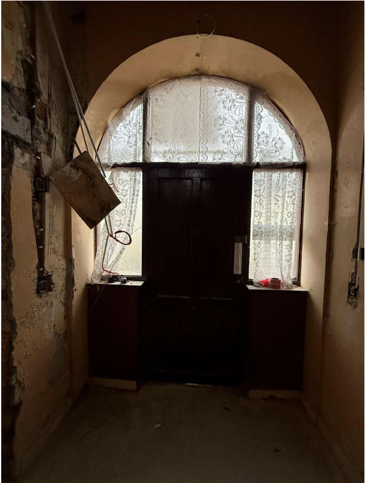
Fig. 9 Interior of front entrance
