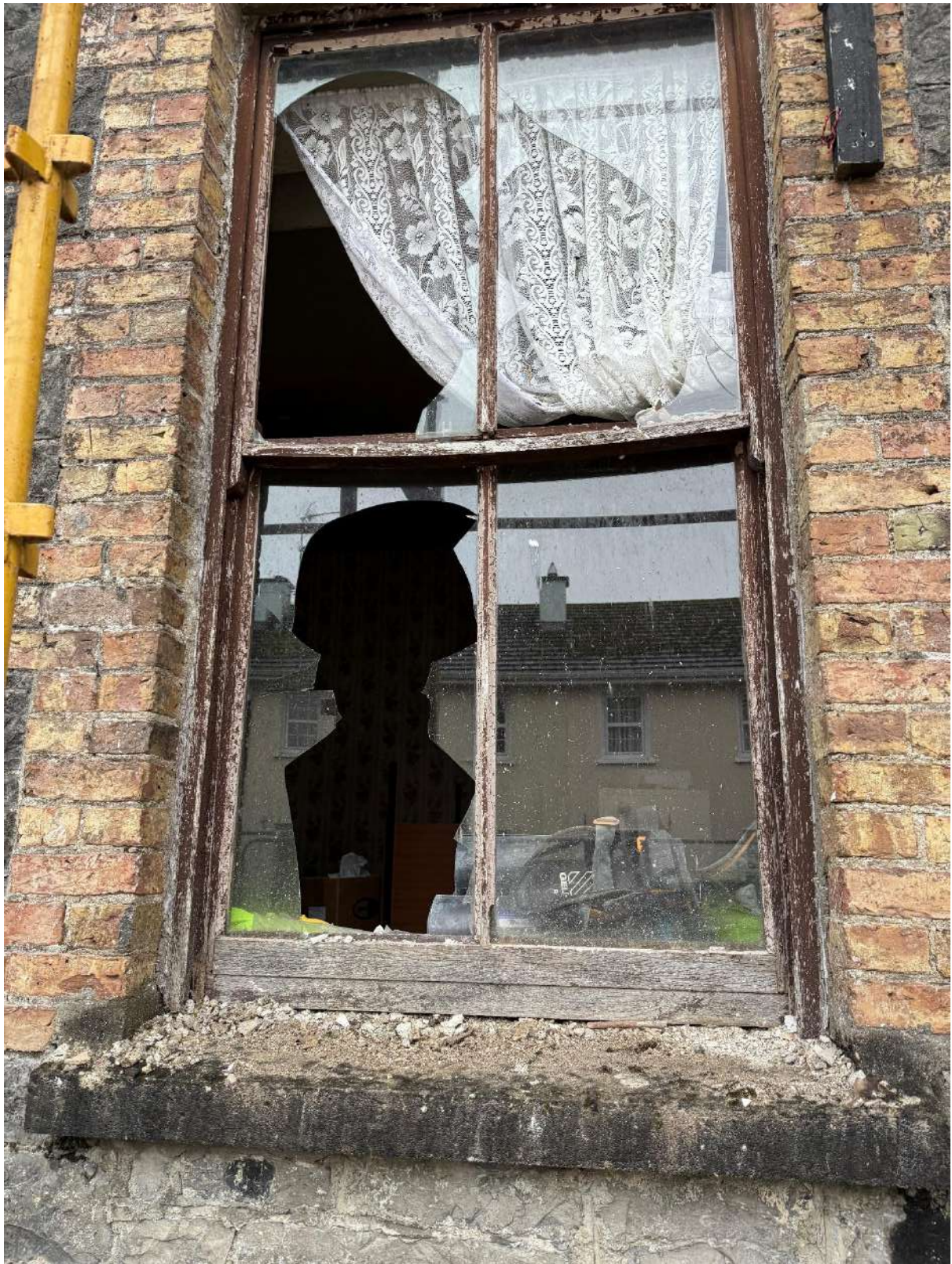
Fig. 7 Replacement timber framed windows to front facade
