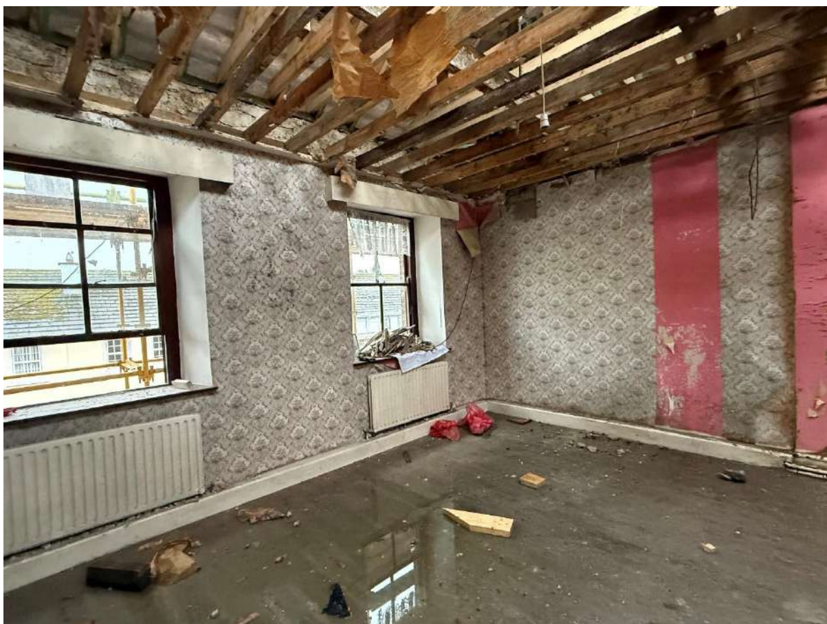
Fig. 13 First Floor interior of room showing ceilings removed
