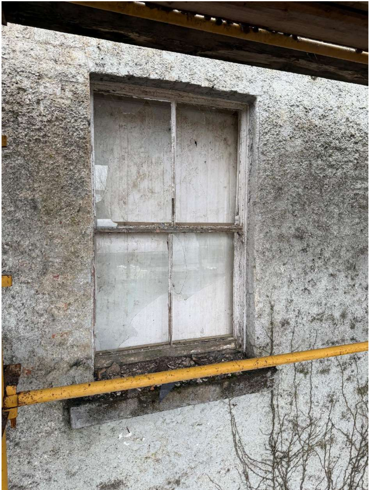
Fig. 8 Surviving two over two timber framed sash window to rear facade
