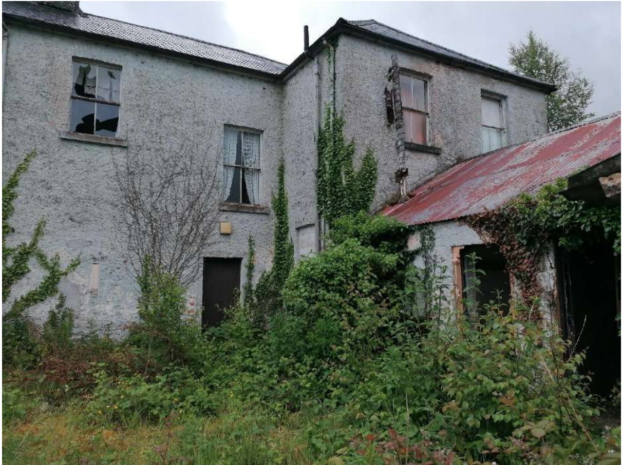
Fig. 4 Rear (North West) elevation
