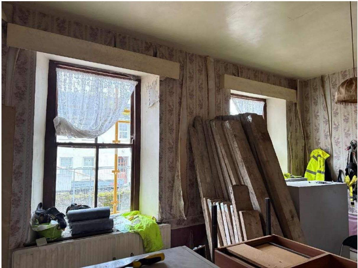
Fig. 12 Typical interior of room showing non-original ceilings & joinery
