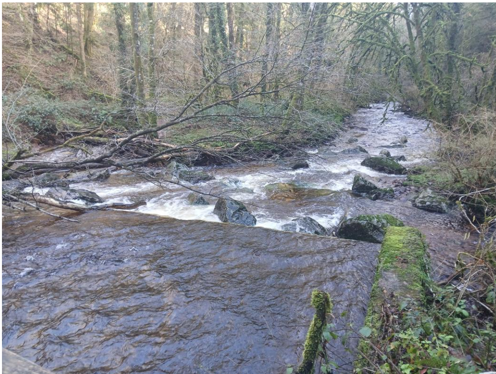
Plate 2 Lyre Bridge – Upstream
