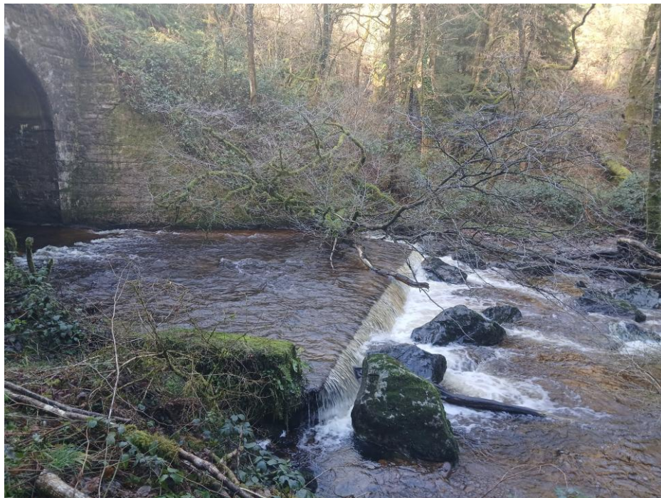
Plate 1 Lyre Bridge - Downstream
