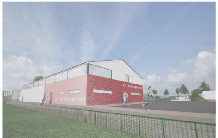
Sports Hall from South-East
