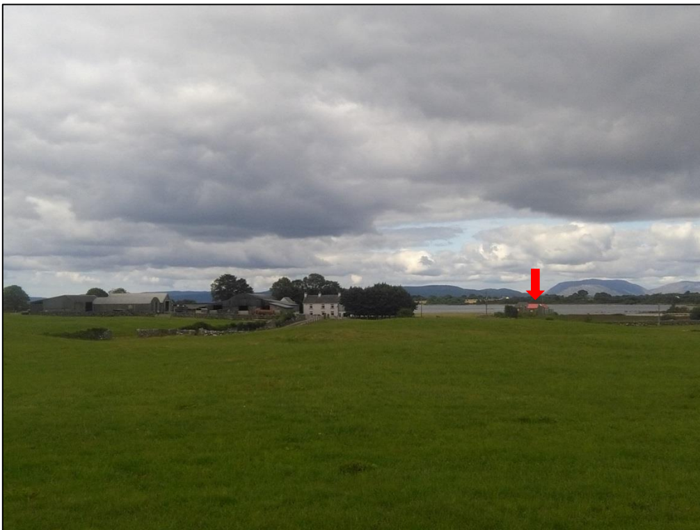
Figure 1: Top – Glencorrib GWS treatment plant facing west towards the main body of the Lough Corrib upper basin; Bottom – The location of the treatment plant (and abstraction point) and the close proximity of a local farm.
