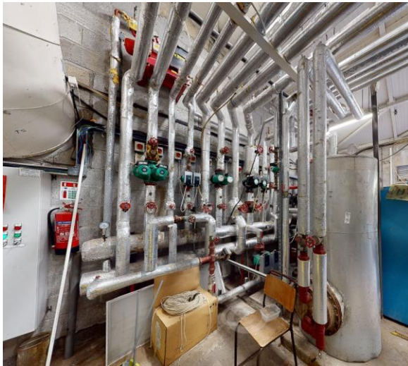
Figure A.7. SRSC – LPHW pipework
