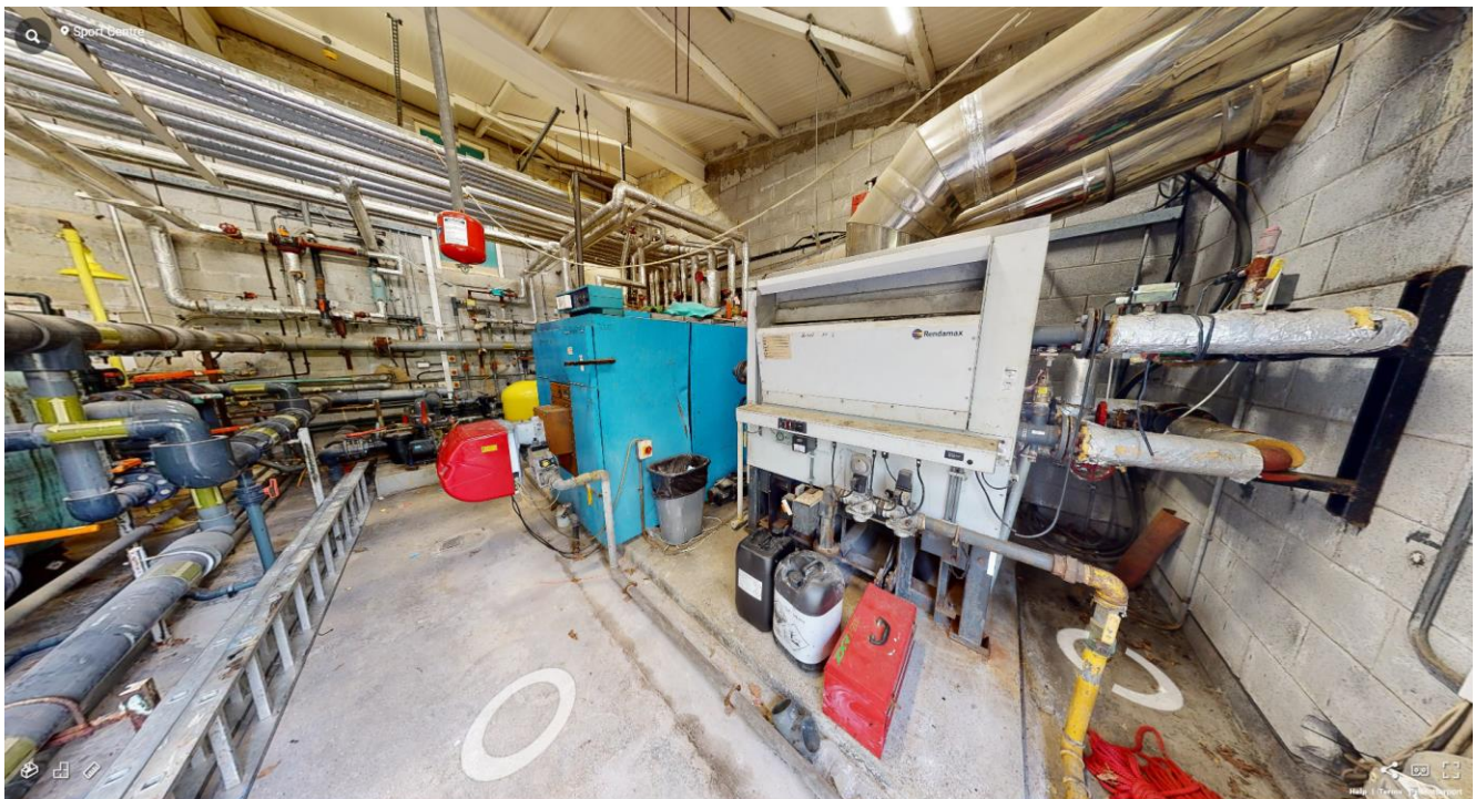
Figure A.5. SRSC – Internal plant room condition
