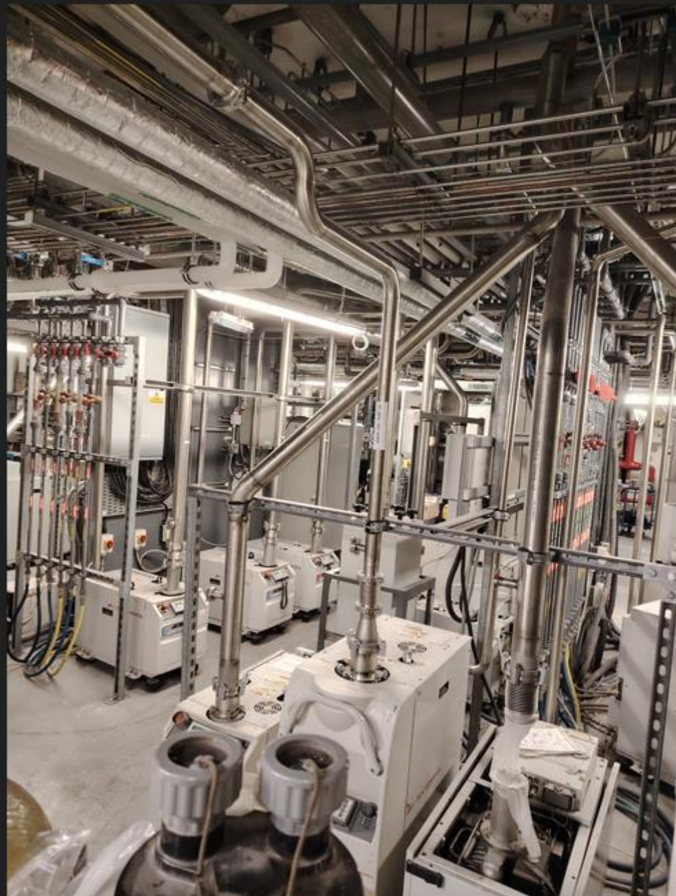
Tyndall Sub-Fab etch & PECVD vacuum-pumps A.png
