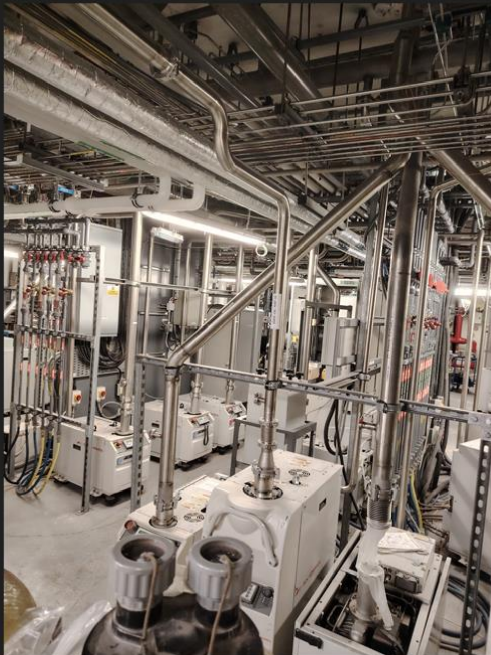
Tyndall Sub-Fab etch & PECVD vacuum-pumps A.png
