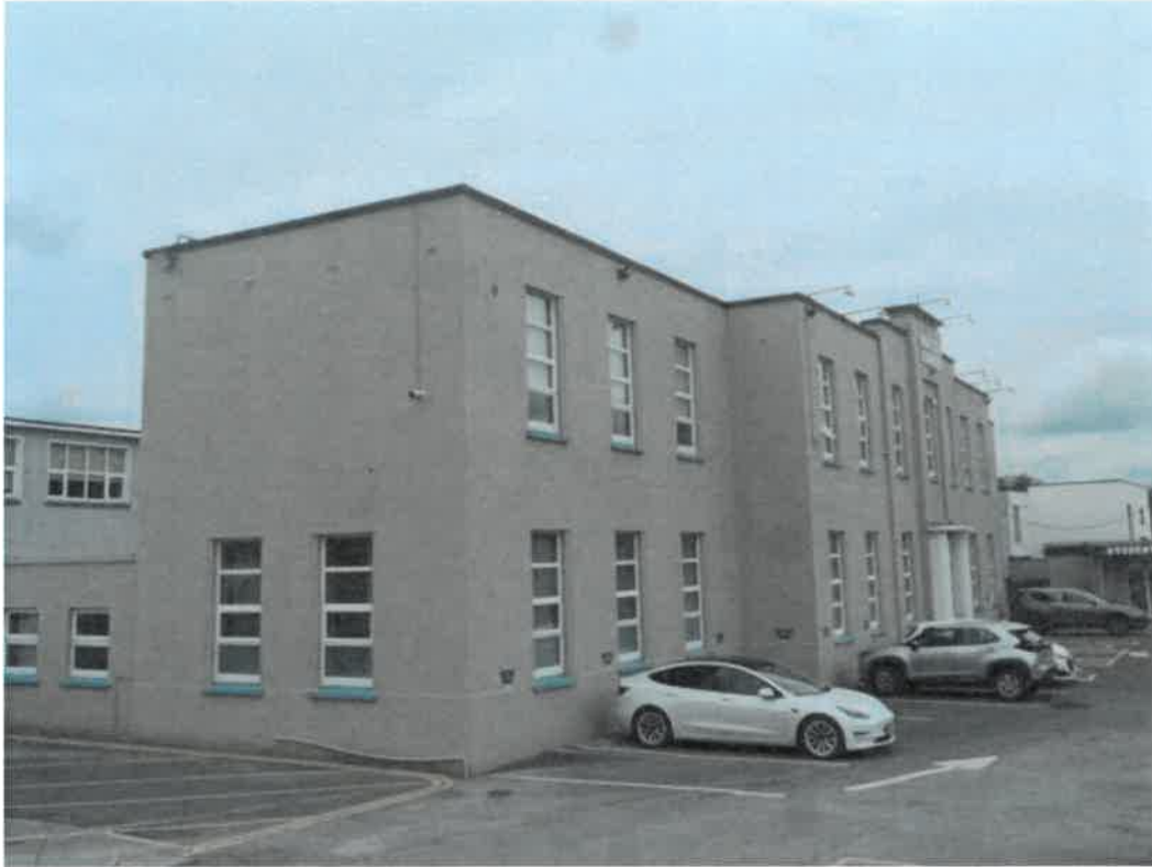
View of Building Block to be worked on
