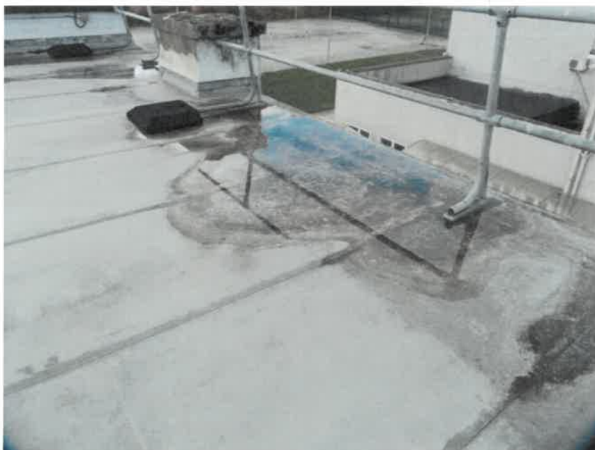
View of ponding & temporary flat roof edge protection
