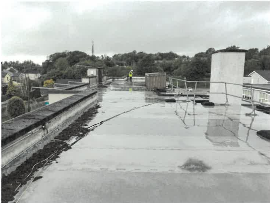
View of roof to be relined
