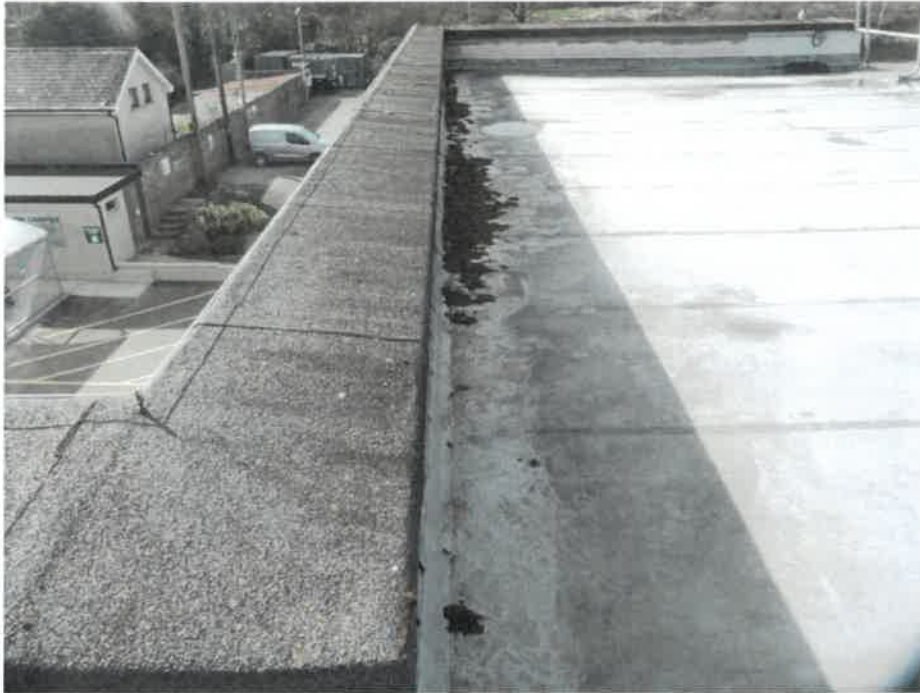
View of present roof lining
