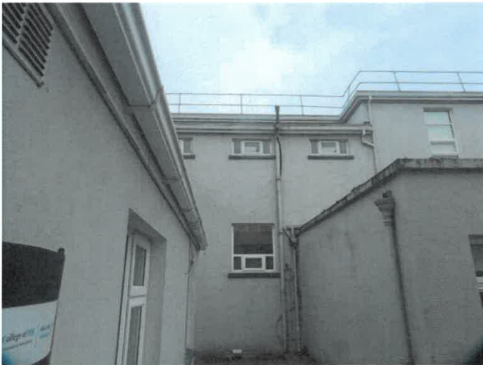
View of building to the rear with temporary flat roof edge protection visible.
