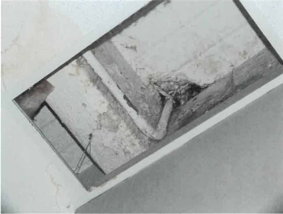
View of underside of roof hard deck from inside
