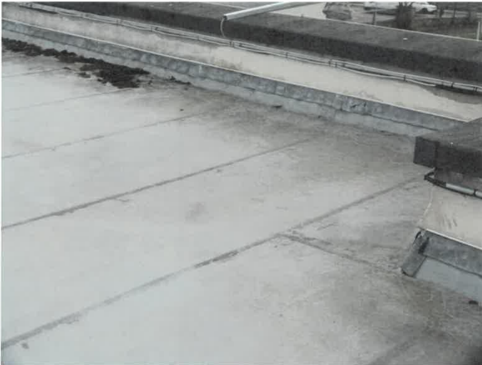
View of existing roof. Single Ply PVC
