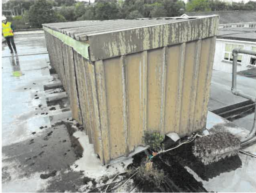
Second view of tank to be removed
