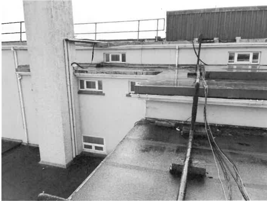
Pipe work to be taken down and disposed of
