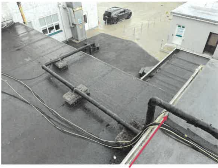
To be removed in total
