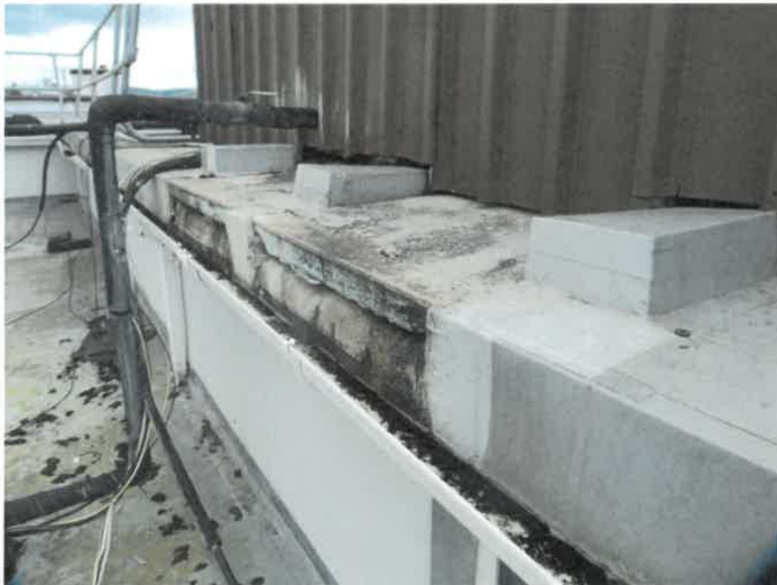
View of water tank to be removed with stubs clearly visible. Stubs and tank to be removed along with pipe work from tank.
