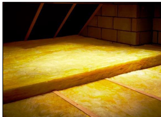
Figure 24: Attic insulation at Ceiling Level
