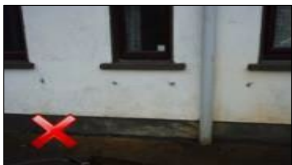
Figure 15: Drill Holes finish details not to standard
